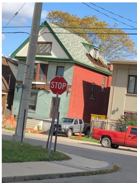
144 Wellington Street North (Before) Source: Applicant
