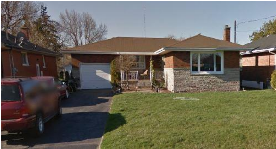
Figure 3 – street view of 7 Pleasant Ave , a single detached brick dwelling.
