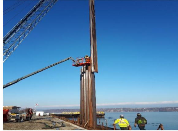
Pier 8 Shorewall Reconstruction
