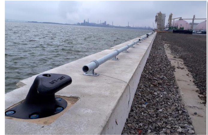
Waterfront Shore Wall Construction
