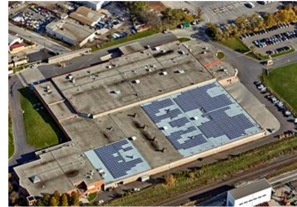
Solar panels-Wentworth Operations Centre
