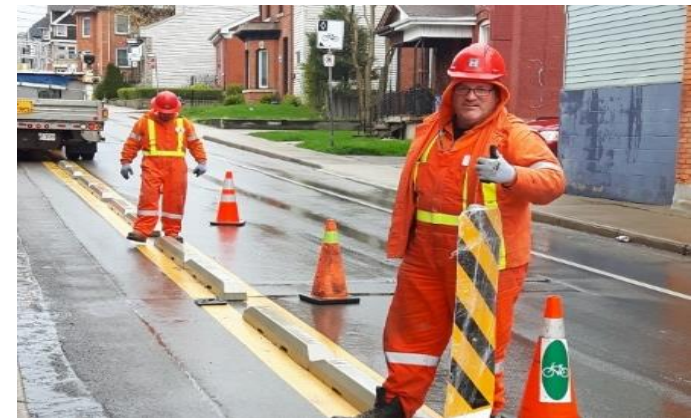
Concrete cycling curbs
