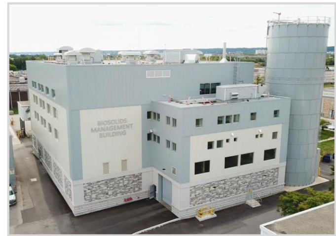
Biosolids Management Facility 16
