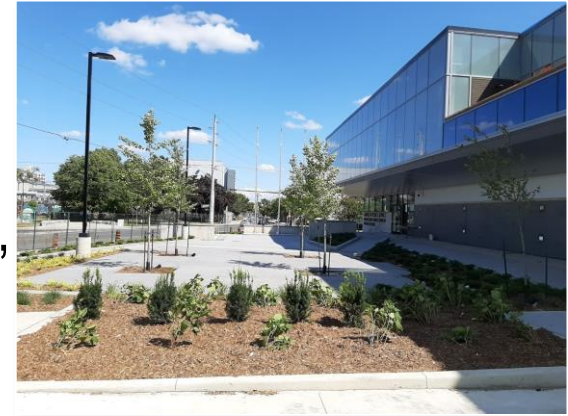
Police Forensics Building
