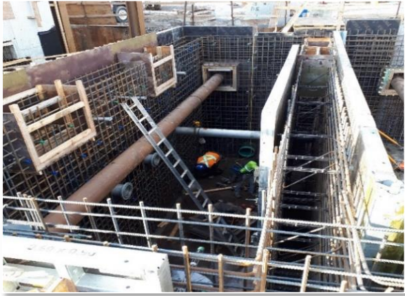
Pier 8 Wastewater Pumping Station
