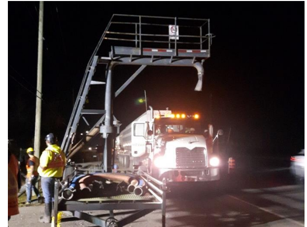
AEGD English church pumping station
