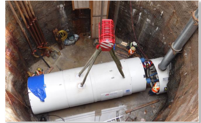
Upper Centennial Parkway Trunk Sewer Project
