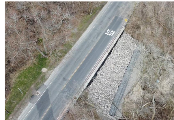
Hwy 8 Dundas Escarpment Repair
