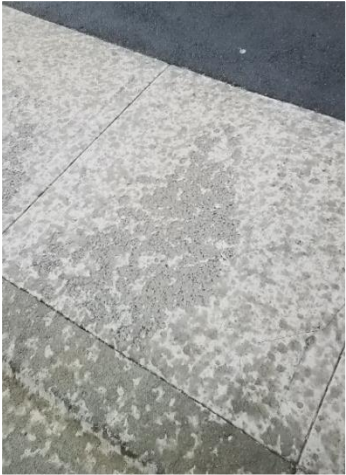
Concrete Spalling
