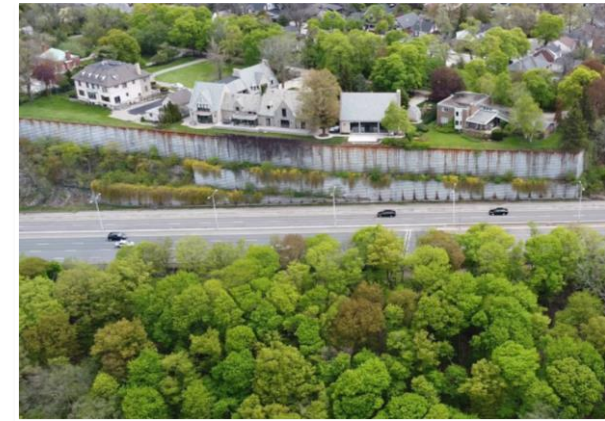
Claremont access bin walls
