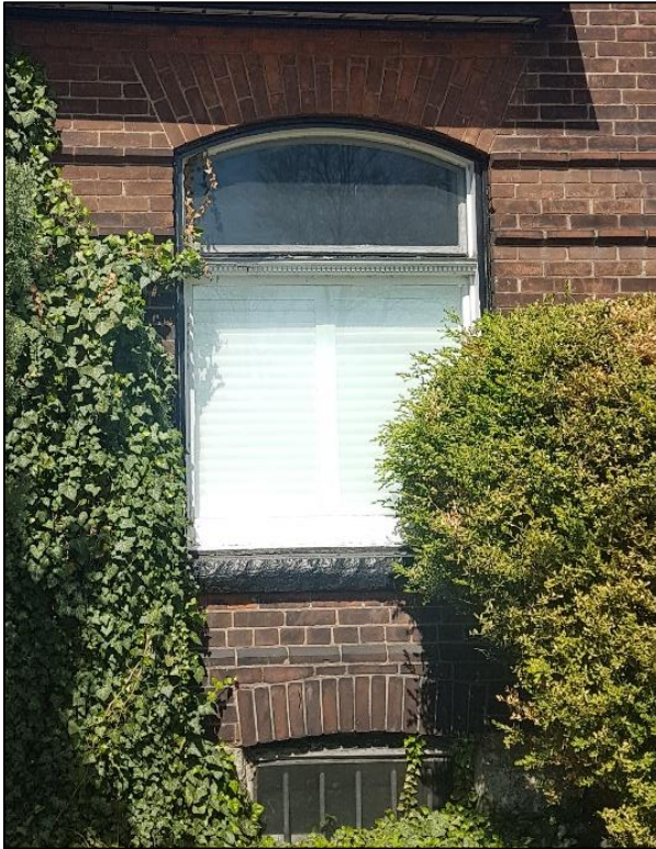
Figure 13: Detail of the fenestration on the front elevation (ASI 2020)
