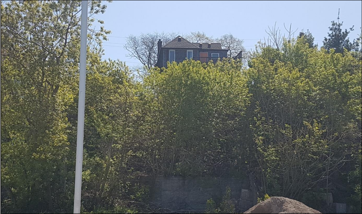
Figure 27: 449 Bay Street North, rear elevation (ASI 2020)
