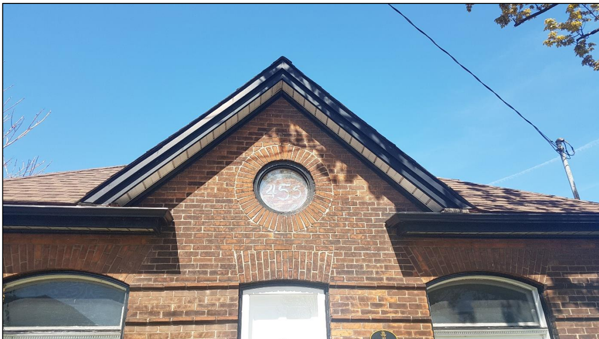
Figure 12: Detail of the centre gable with circular window (ASI 2020)
