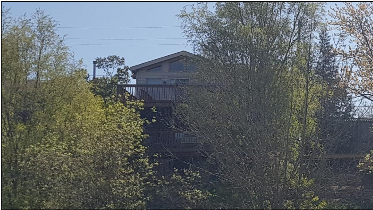
Figure 29: 459 Bay Street North, rear elevation (ASI 2020)
