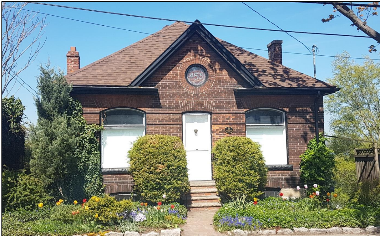
Figure 11: 455 Bay Street North, front elevation (ASI 2020)
