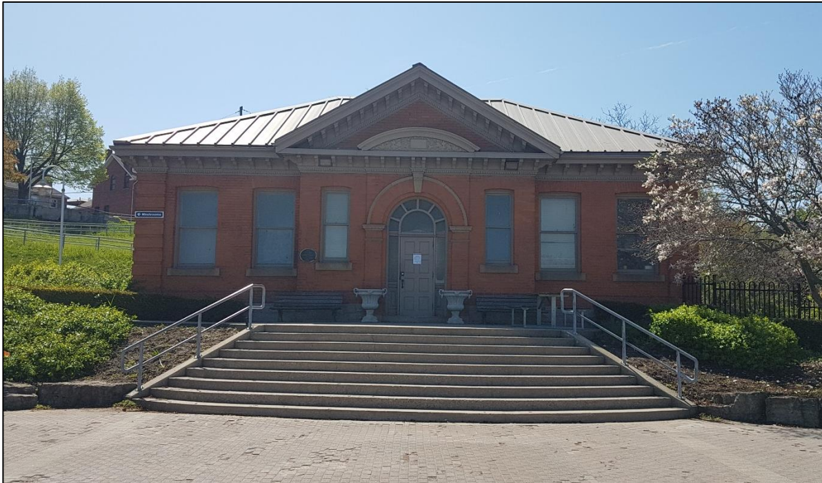
Figure 30: Gartshore-Thomson Building (ASI 2020)
