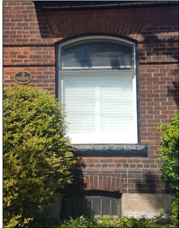
Figure 14: Detail of the fenestration on the front elevation (ASI 2020)
