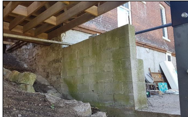
Figure 23: Wooden deck, concrete block wall and poured concrete behind the residence (ASI 2020)
