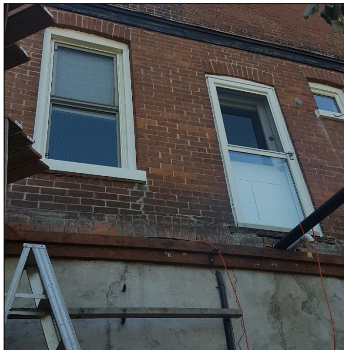
Figure 20: Detail of the rear entrance, window and foundation (ASI 2020)
