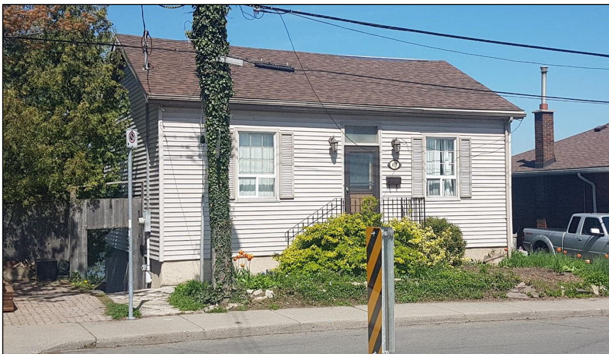
Figure 28: 459 Bay Street North (ASI 2020)
