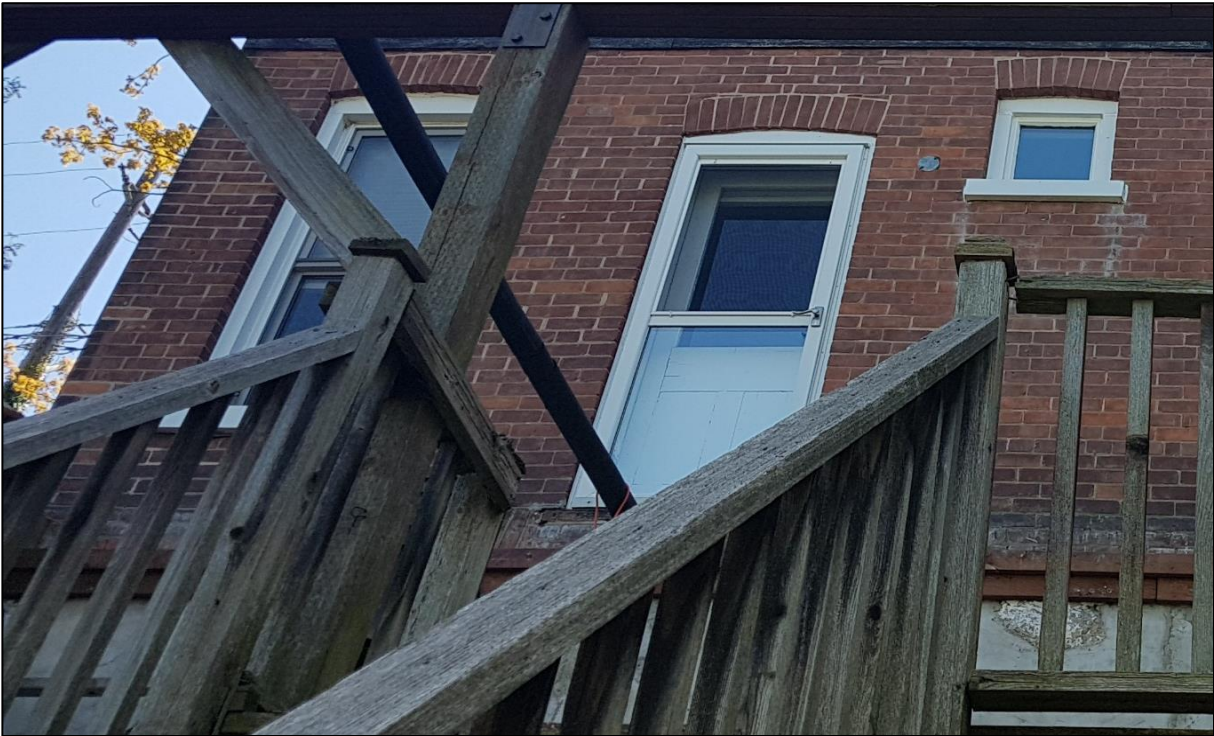
Figure 19: Detail of the rear entrance (ASI 2020)
