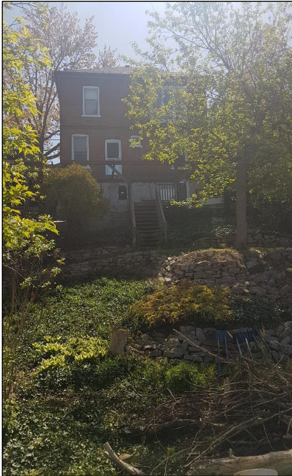
Figure 22: Rear of the property showing the slope (ASI 2020)
