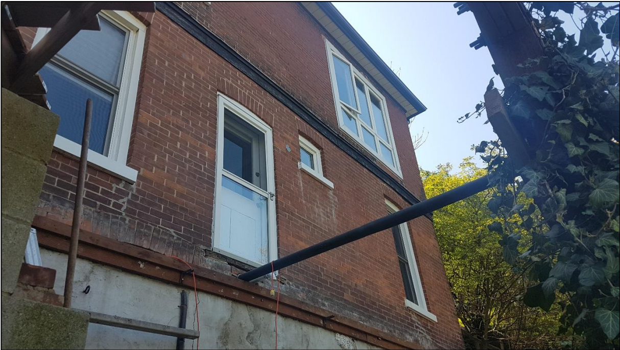
Figure 18: Detail of the rear elevation (ASI 2020)
