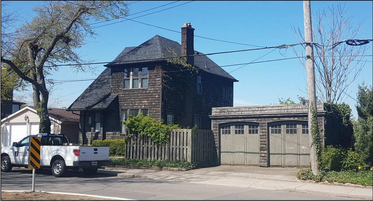
Figure 26: 449 Bay Street North, front elevation (ASI 2020)
