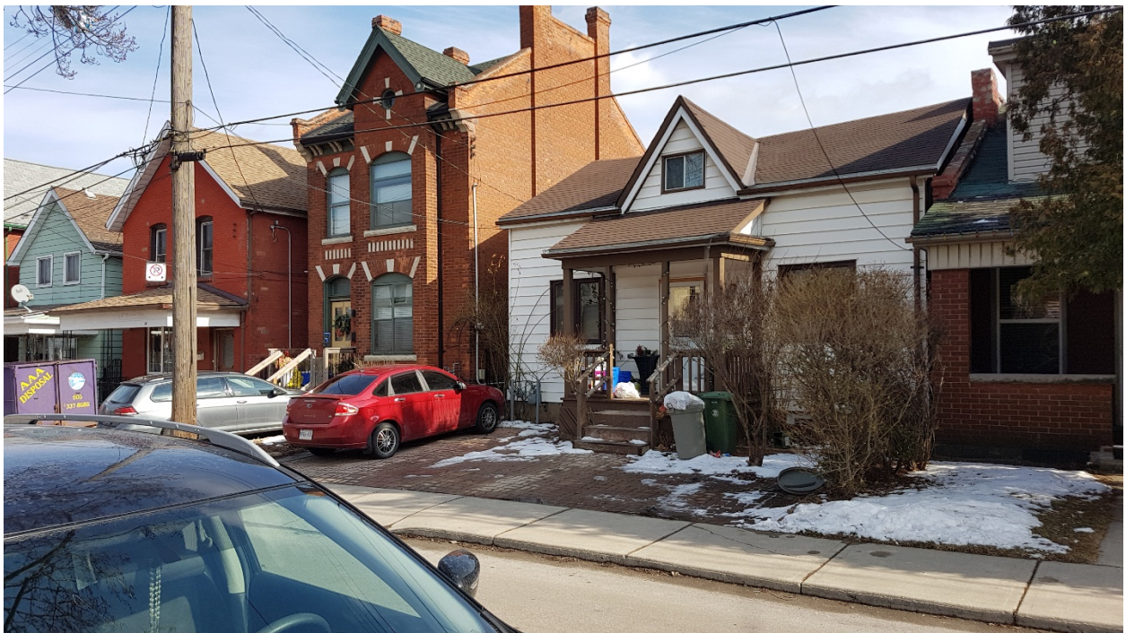
Images of other housing units on Magill Street. 51 and 53 Magill Street.
