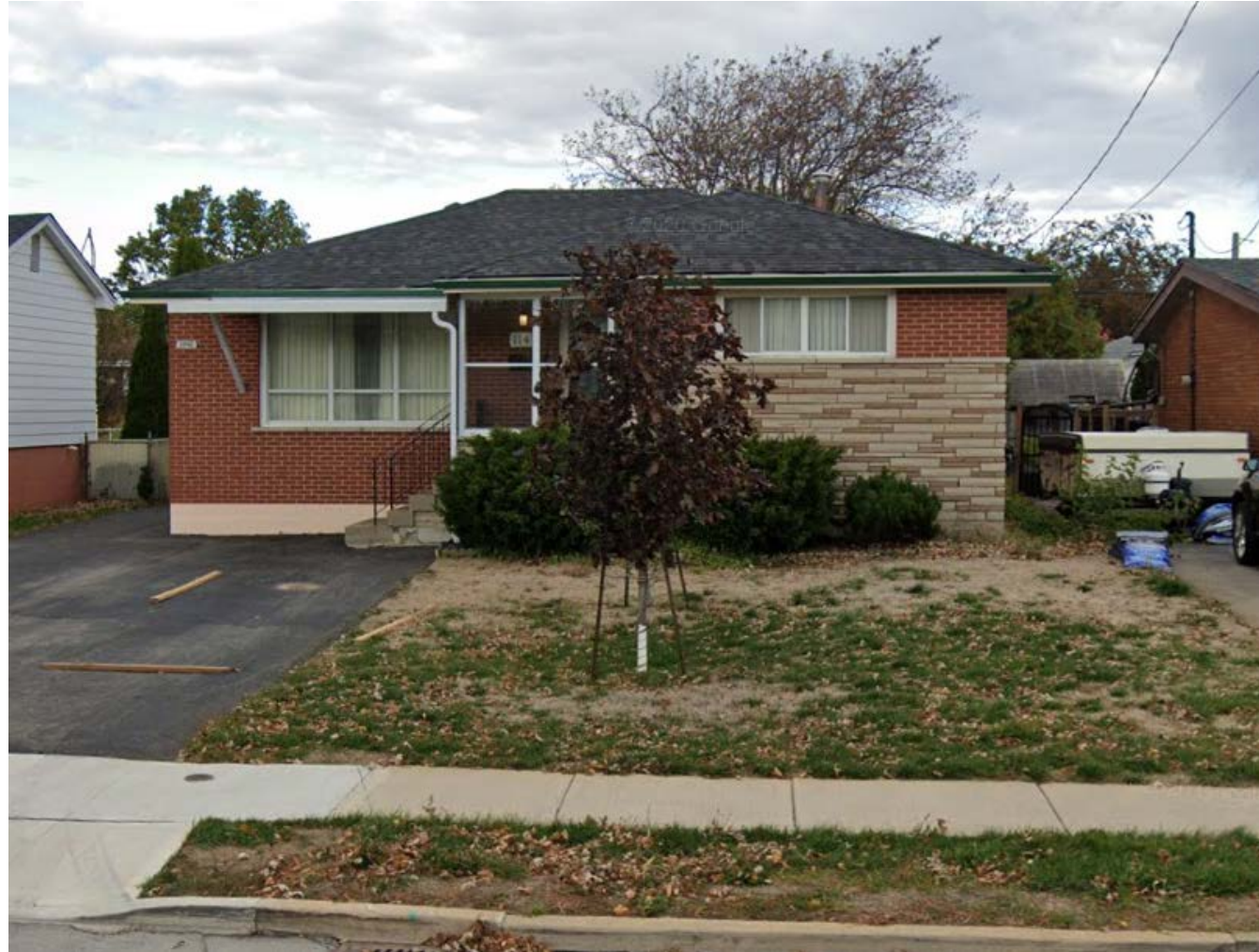
EXISTING BUILDING IMAGE
