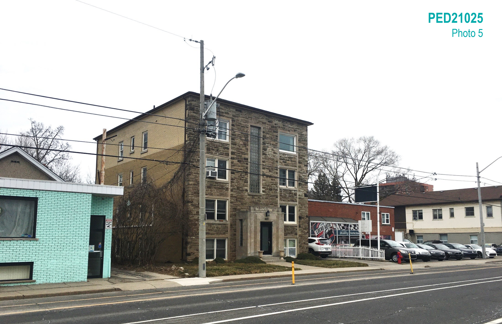
Existing development to the east, as seen from King Street West
