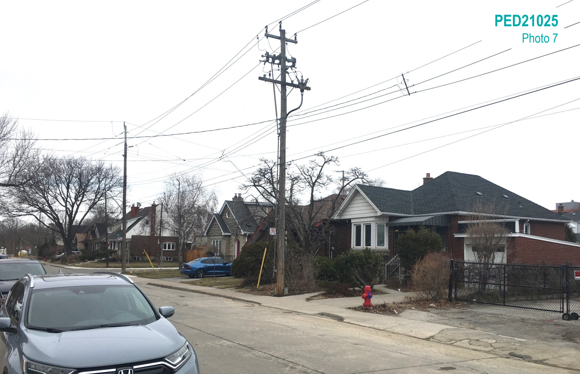
Existing development to the north, as seen from Paradise Road North
