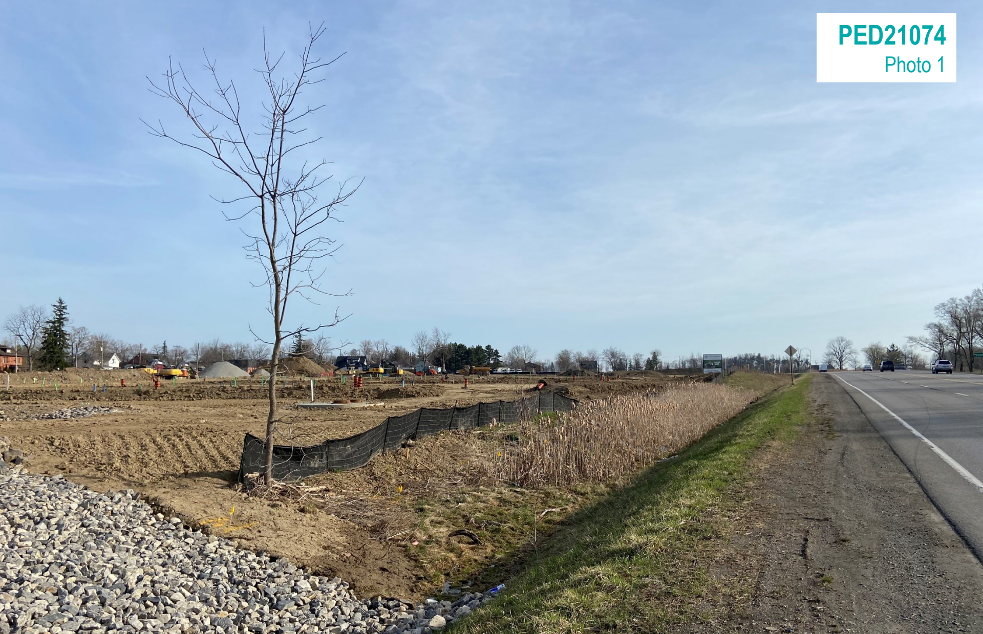
Site view from South East Corner
