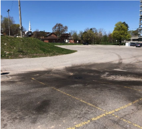
Oil Spill at 200 Market St parking lot.
