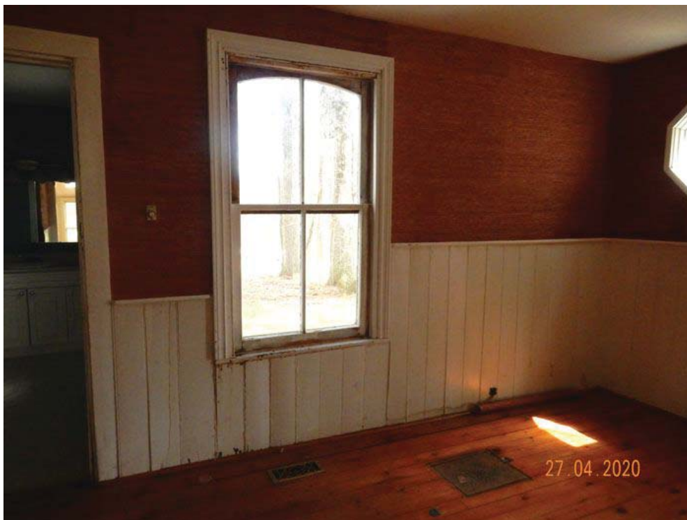
Figure 9: Interior Rear Addition, 1389 Progreston Road
