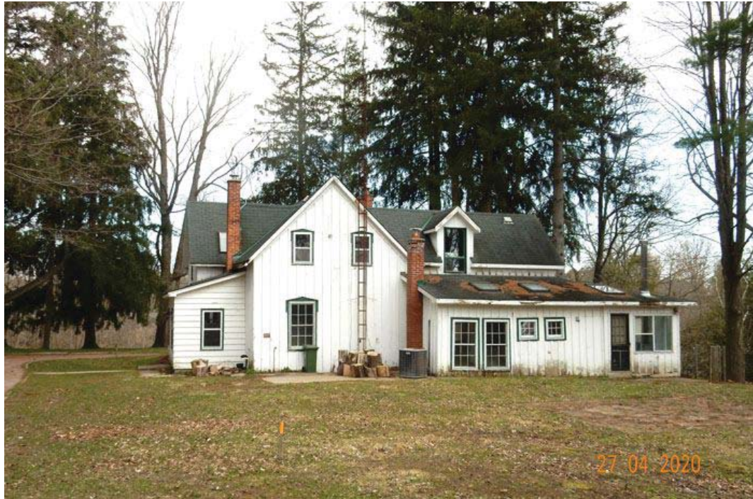
Figure 2: Rear Elevation, 1389 Progreston Road
