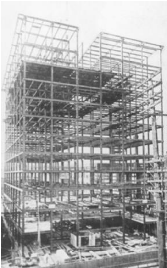
Left: 1914-16 building steel frame under construction; Right: 1931 building under construction. Image source: PreView Image Database, Hamilton Public Library, www.preview.hpl.ca .
