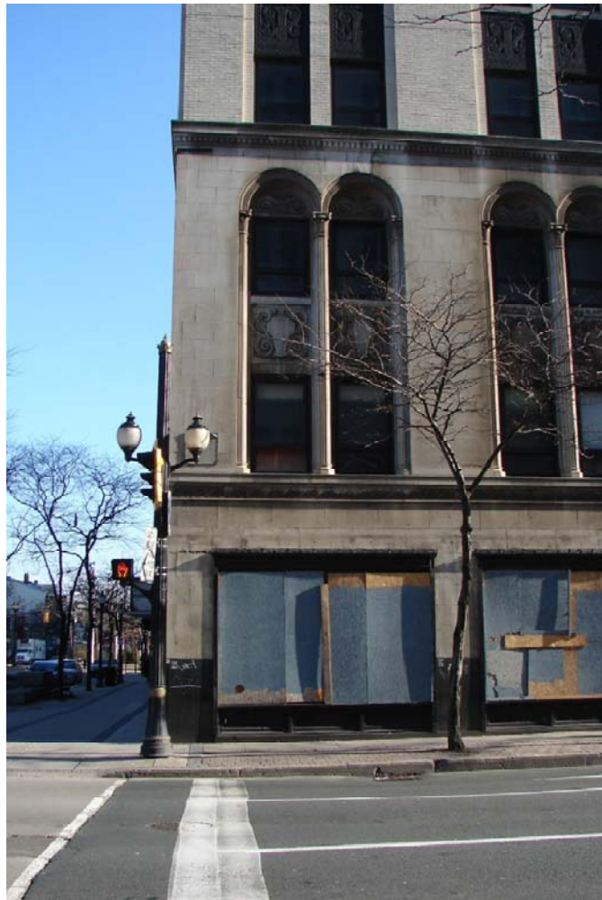
Fig. 71 Bays nearest King Street East on west elevation's base
