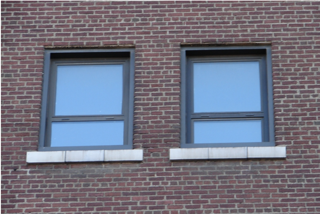
Fig. 48 Pair of windows in shaft
