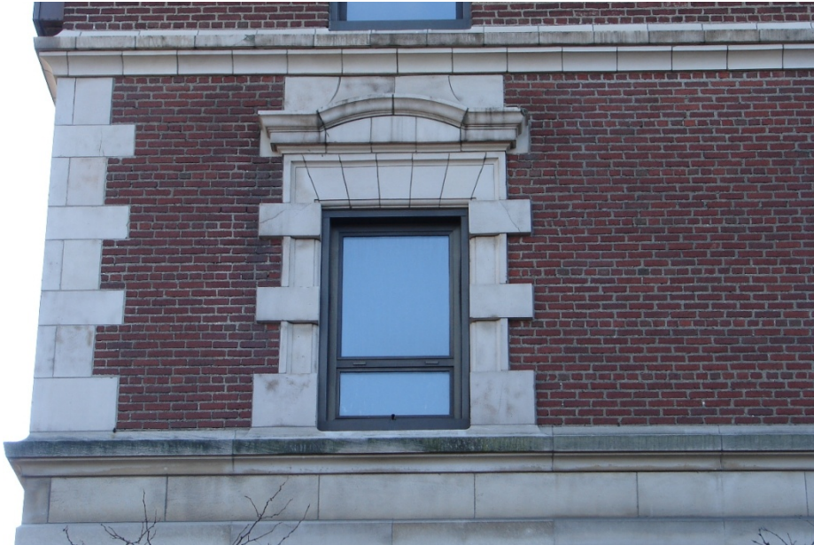
Fig. 46 Second-floor window with terra cotta surrounds
