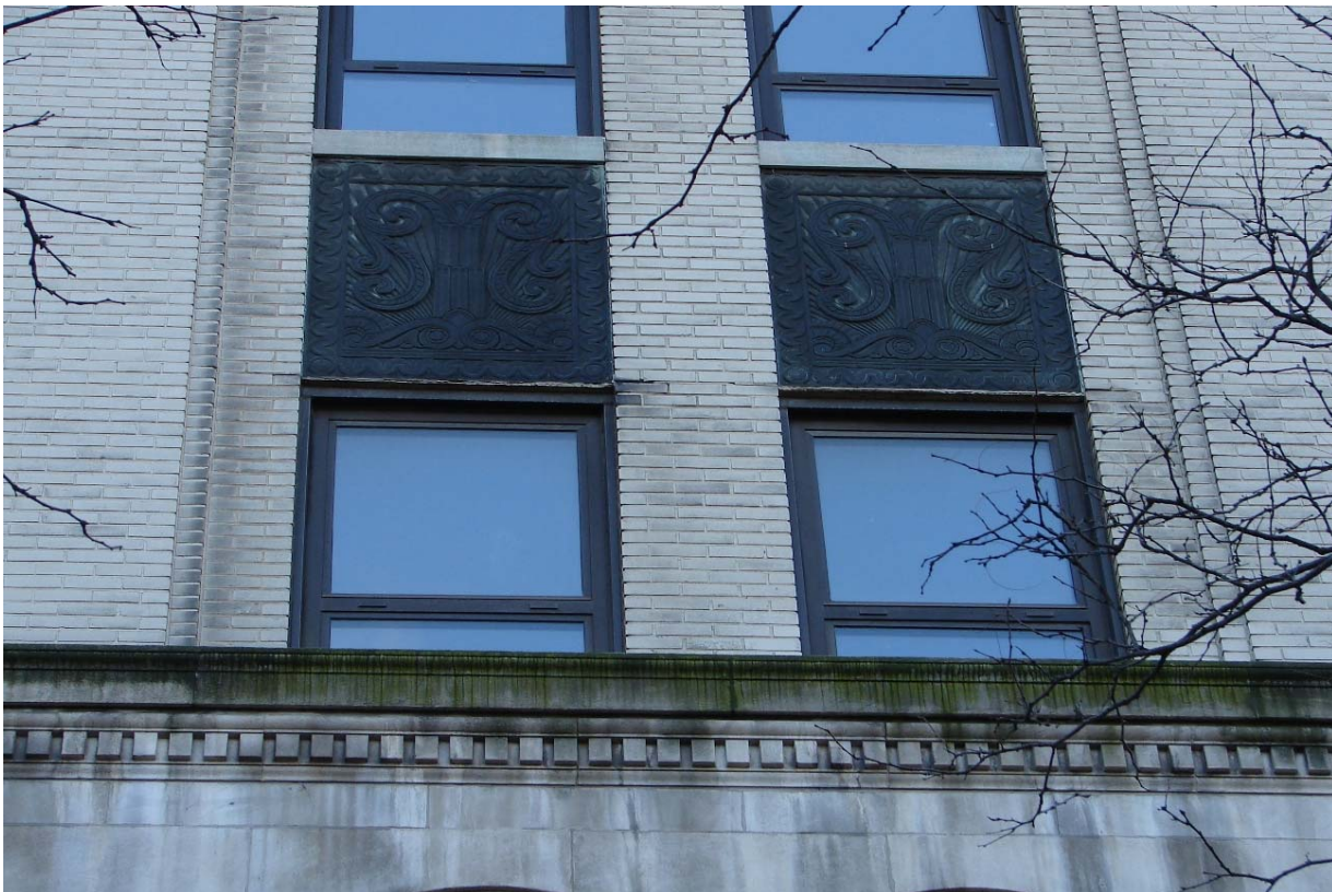
Fig. 57 Windows in shaft
