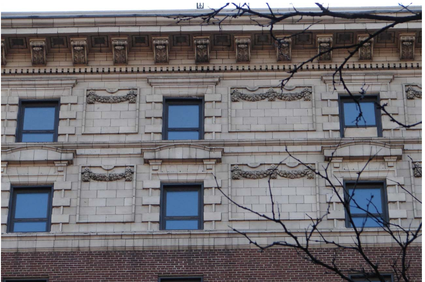
Fig. 49 Detail of terra cotta upper floors in front facade of Edwardian building
