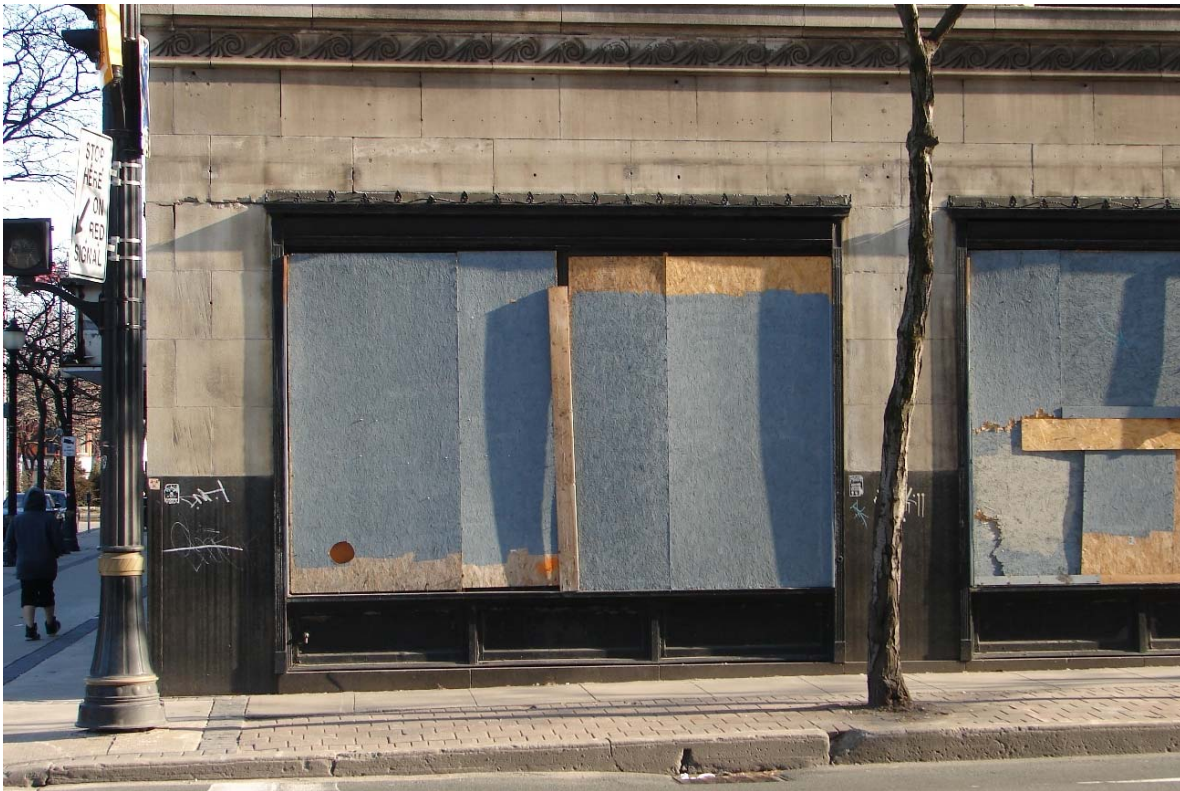
Fig. 72 Storefront in west elevation's ground floor (note also brown polished granite foundation veneer and limestone stringcourse in an Art Deco wave pattern)
