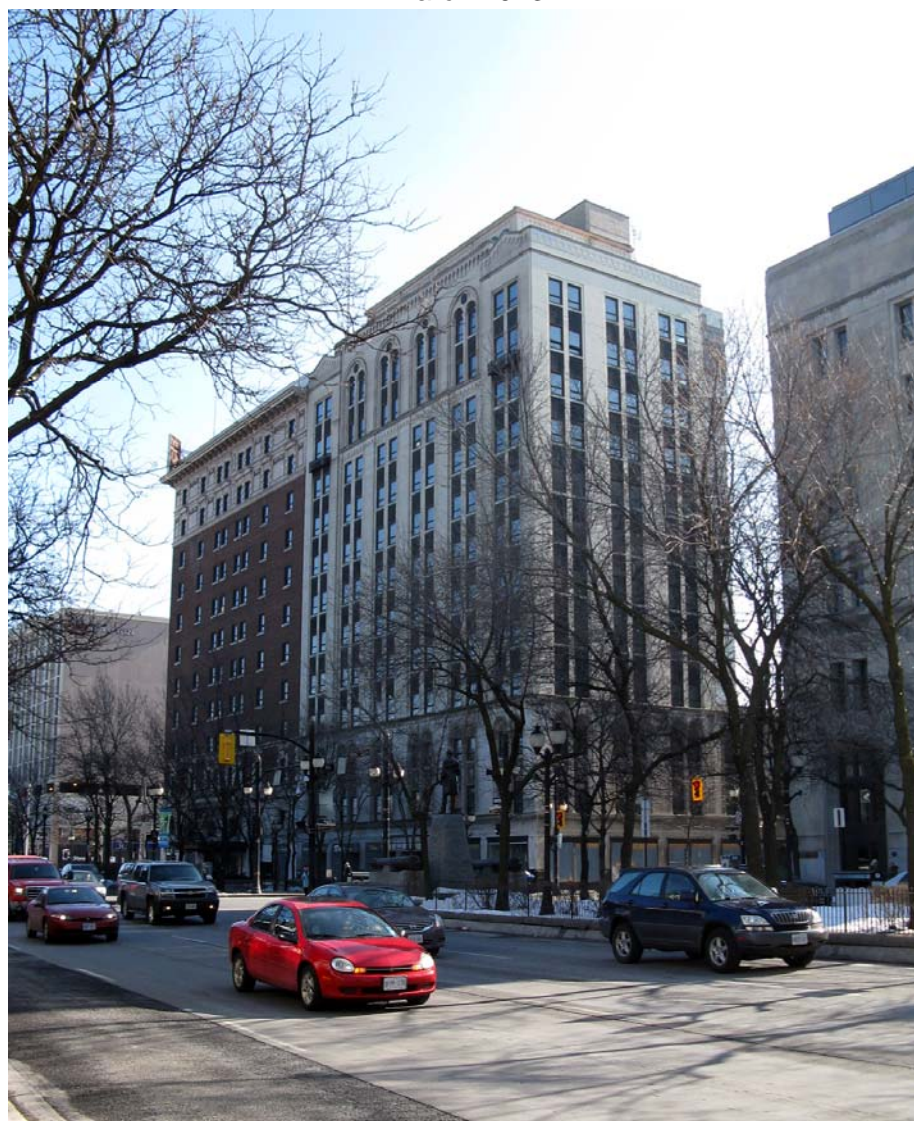
Fig. 1 View of the Royal Connaught Hotel from the northwest
