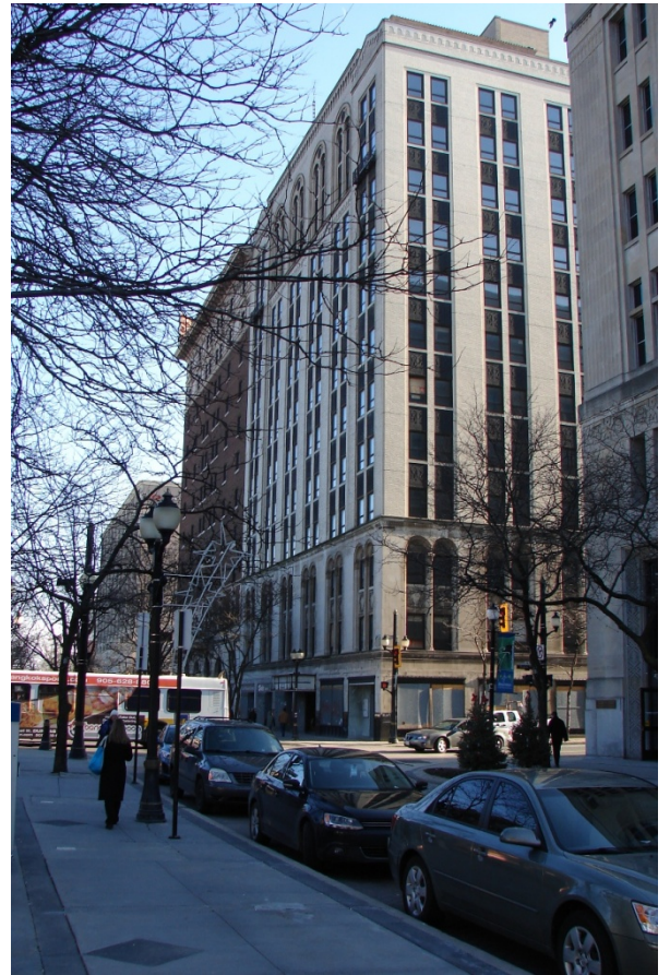
Fig. 31 Corner view of the front facade and west tower's west elevation, looking east from the King Street East island (notice the corner of the old Dominion Public Building on the far right of the frame)
