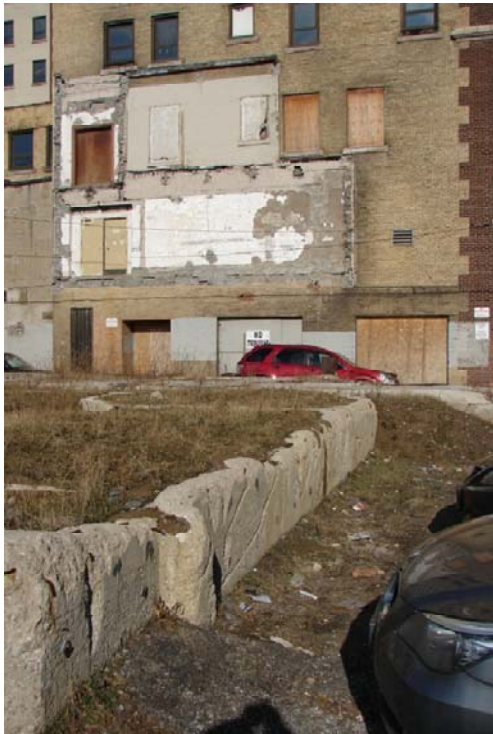
Fig. 78 Concrete foundation wall of former swimming pool
