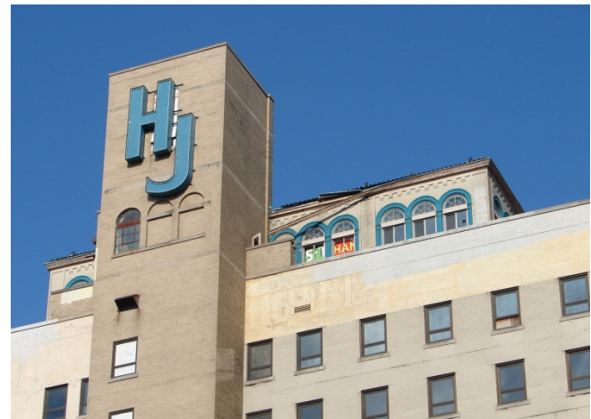
Fig. 77 Top of the rear elevation of Art Deco addition
