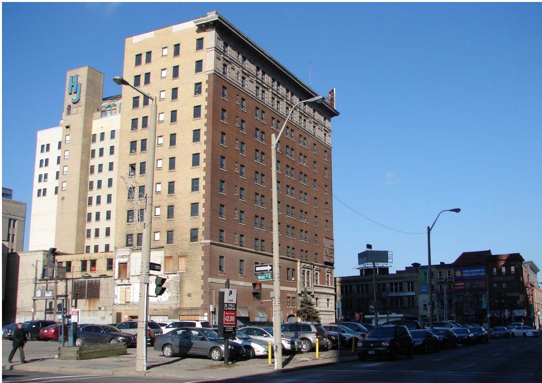
Fig. 38 Corner view of the rear and east elevations from Main Street East and Catharine Street South, looking north to the north side of King Street East
