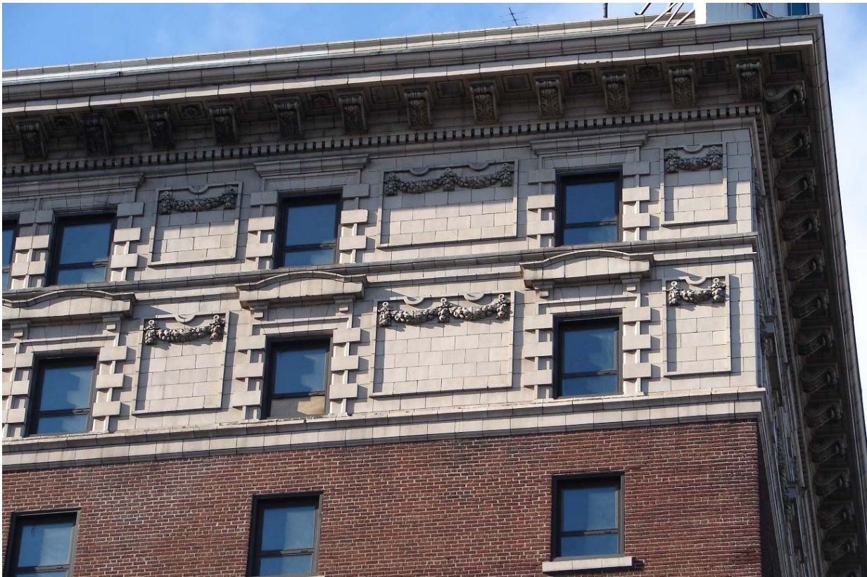
Fig. 68 Detail of upper two floors in terra cotta
