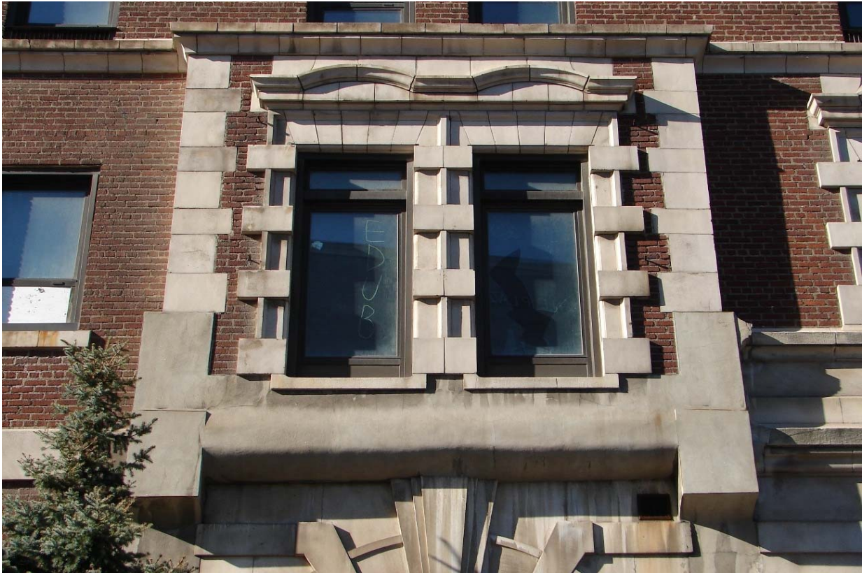
Fig. 67 Oriel window in limestone, terra cotta and rug brick
