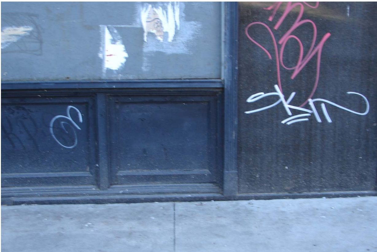
Fig. 53 Detail of metal panels in storefront
