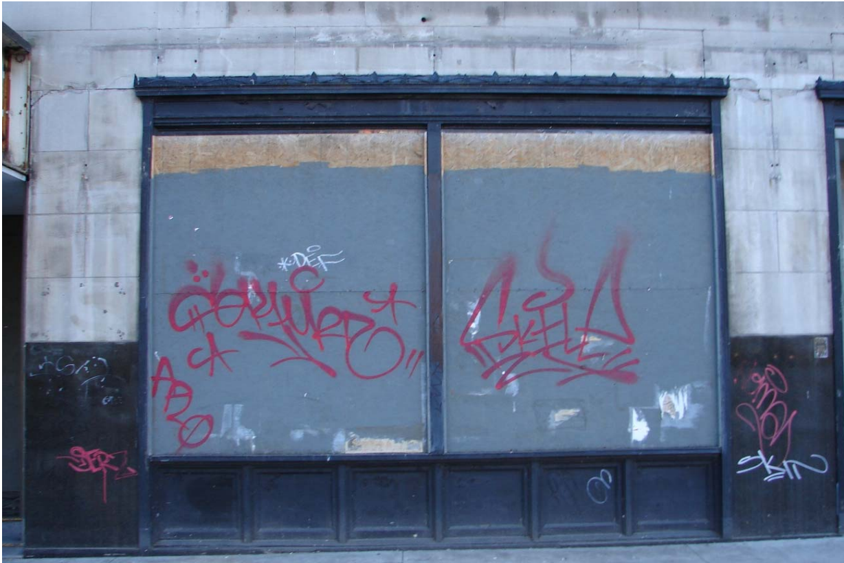
Fig. 52 Typical storefront on ground floor
