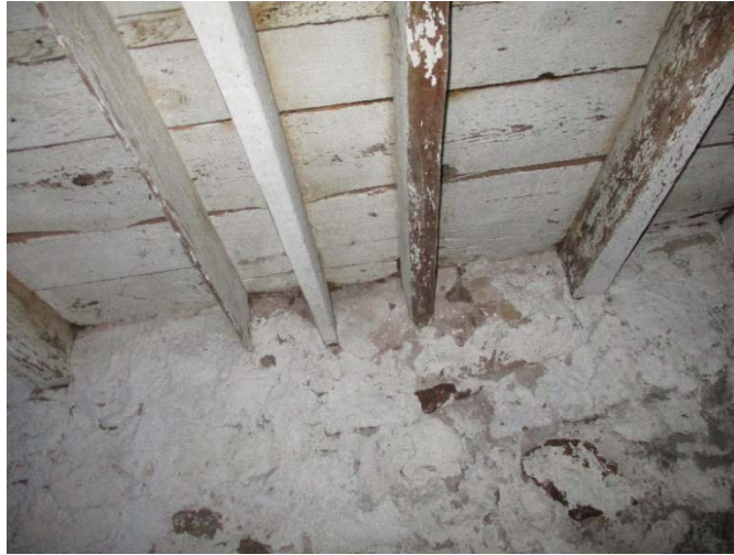
Randomly sized and spaced circular-sawn floor joists
