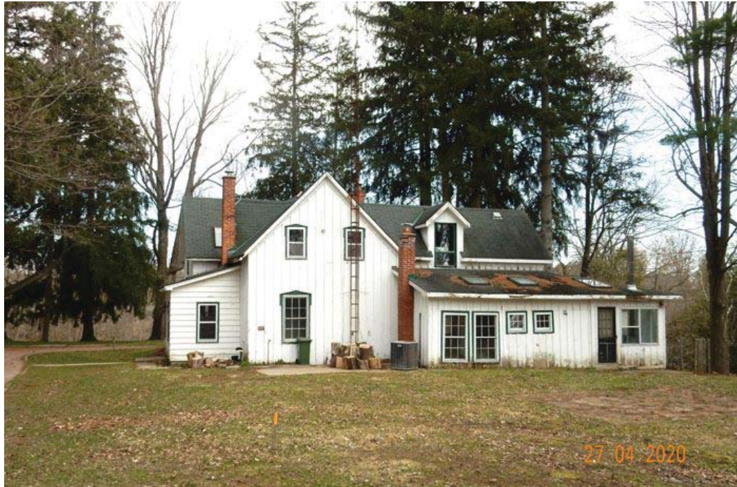
Figure 2: Rear Elevation, 1389 Progreston Road
