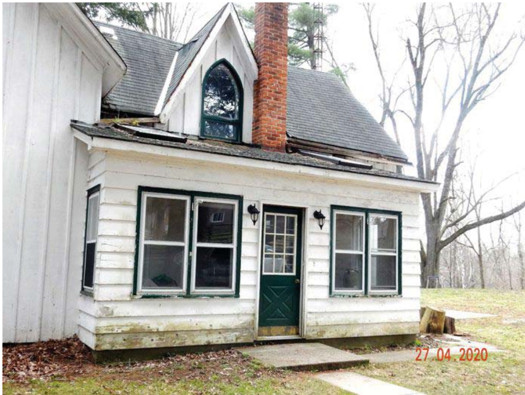
Figure 5: North Elevation, 1389 Progreston Road
