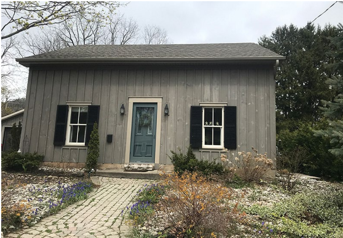
1½ storey frame cottage at 251 MacNab Street with a tall symmetrical façade featuring a simple framed doorway and two two-over-two paned sash windows with wood sills and lintels. View below shows the west side wall and the top of a two-storey rear addition. When built the entire house was reclad in board-and-batten.
