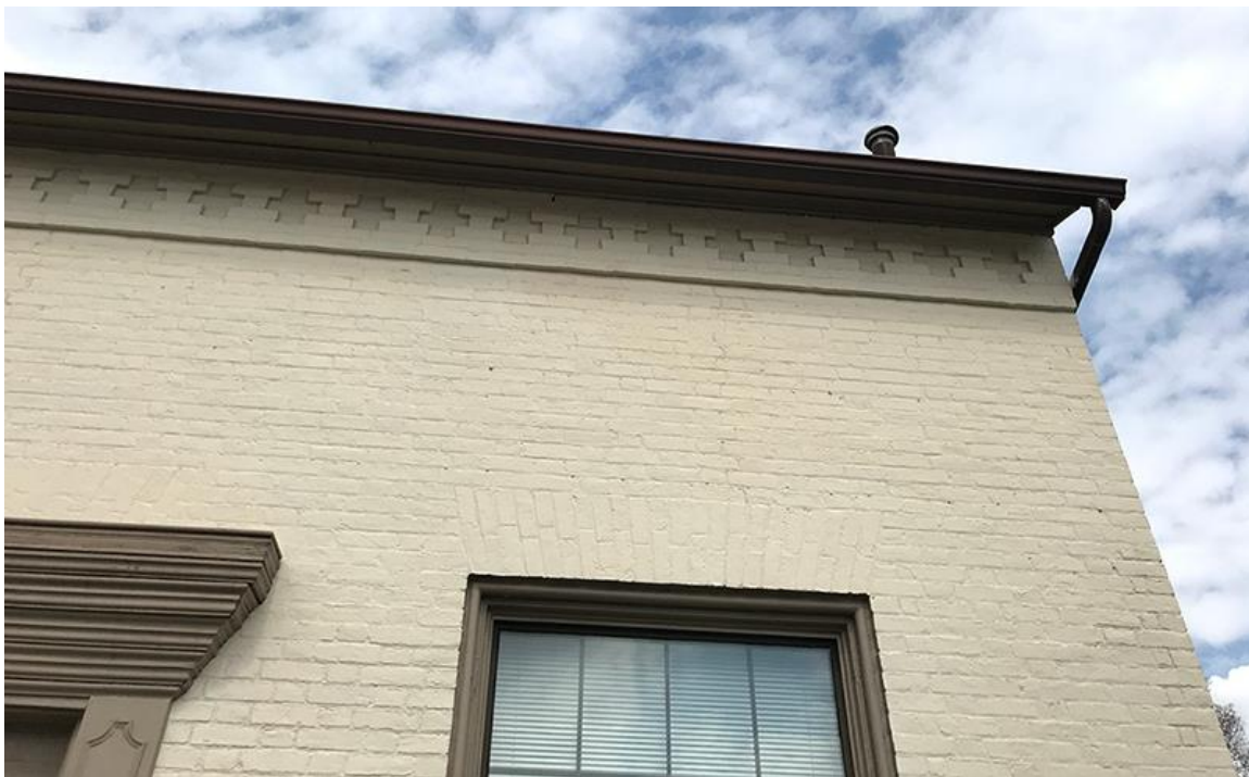
Close-up view of the decorative band of raised brickwork with the cross motif. Also shows the Flemish bond brickwork of the front façade and the flat voussoir arched window and door lintels. The door lintel is largely obscured by the added wood lintel and pilasters. Photo credit: Ann Gillespie, March 2021
