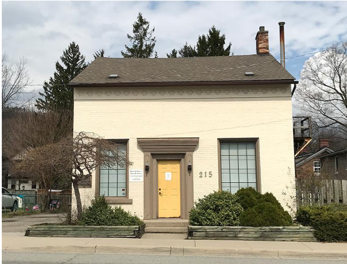
Front (south) façade of #215 showing the decorative course of brickwork below the eaves, and the altered front doorway and windows (thermopane replacements with fake mullions). Photo credit: Ann Gillespie, March 2021
