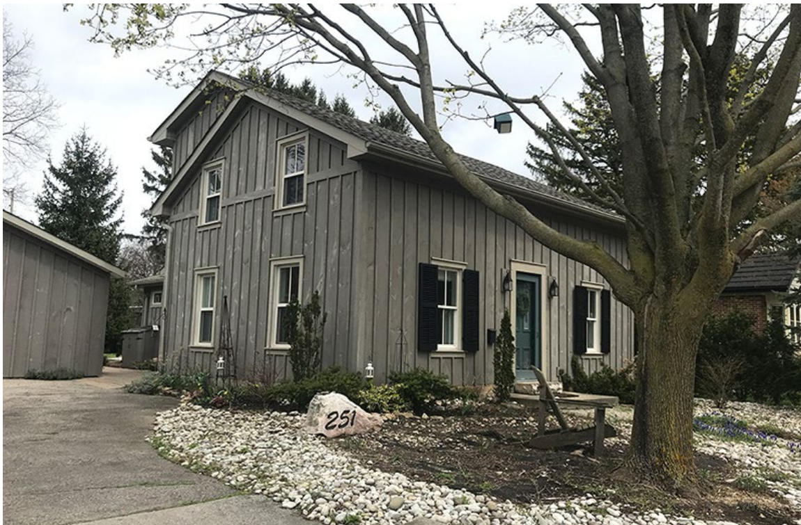
1½ storey frame cottage at 251 MacNab Street with a tall symmetrical façade featuring a simple framed doorway and two two-over-two paned sash windows with wood sills and lintels. View below shows the west side wall and the top of a two-storey rear addition. When built the entire house was reclad in board-and-batten.
