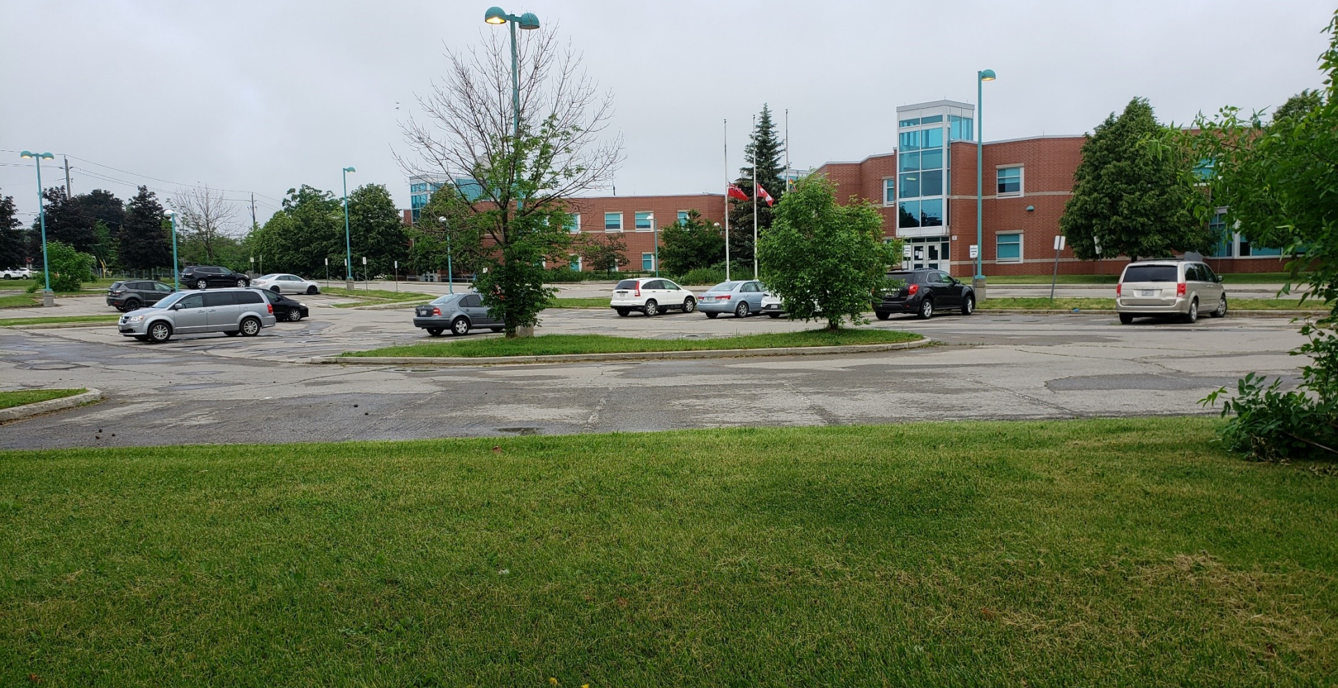
Saltfleet District High School
