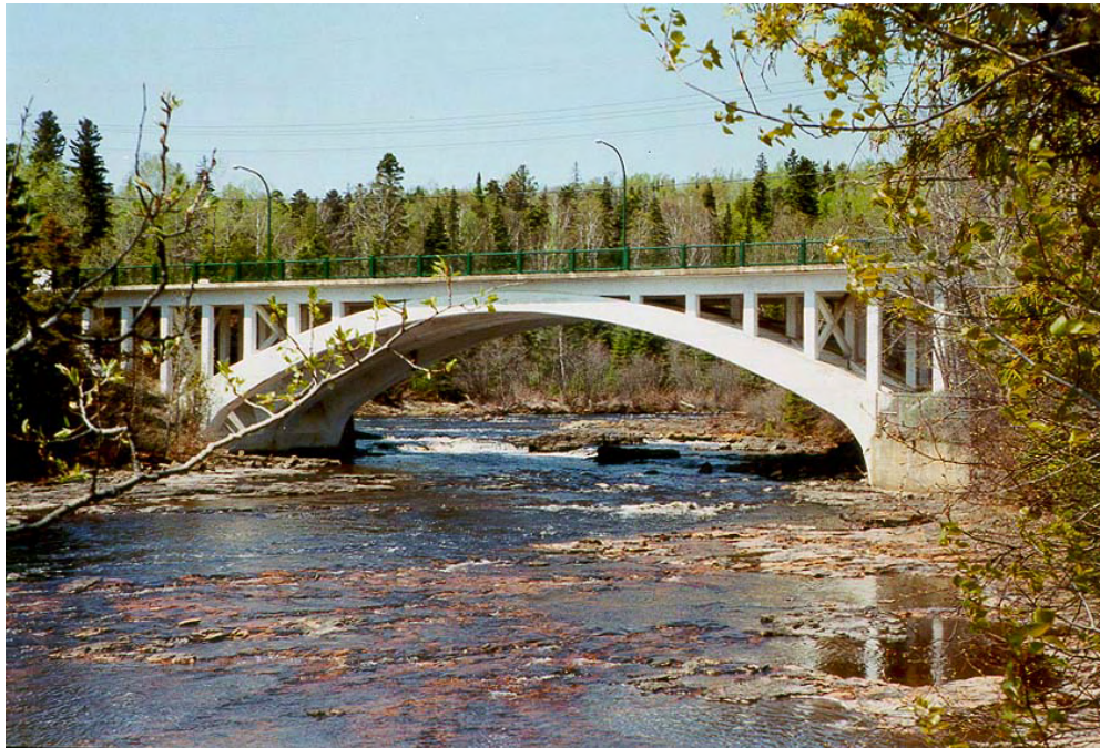
Figure 4. The Black Bay bridge in the city of Thunder Bay was one of the first single spandrel reinforced concrete bridges ever constructed (MHSTCI).
