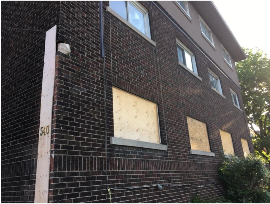
Photo #5 taken June 2019 when building became vacant. Tenants in a Block A move out.
