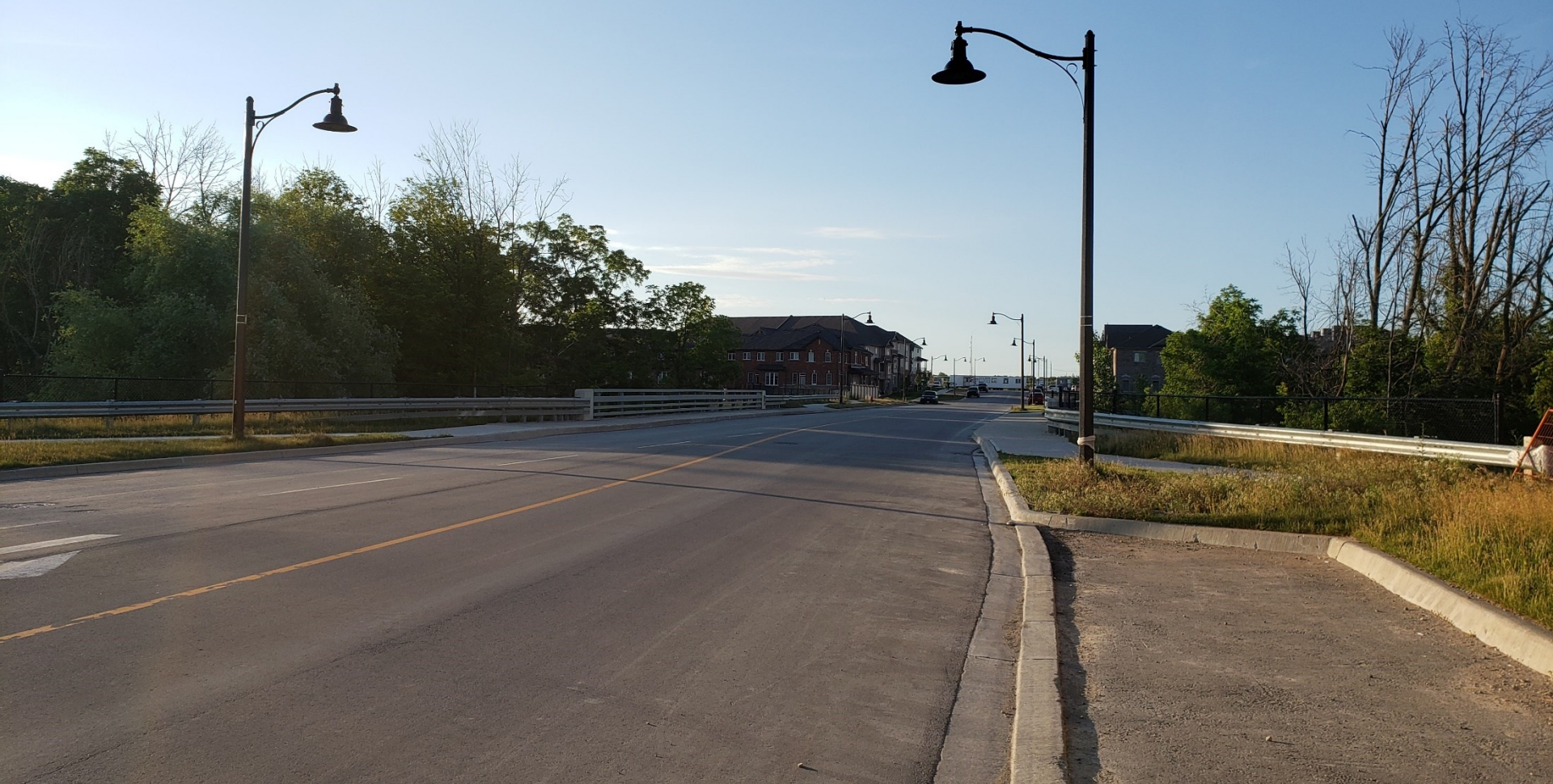
Existing Townhouses and Conservation Lands to the East
