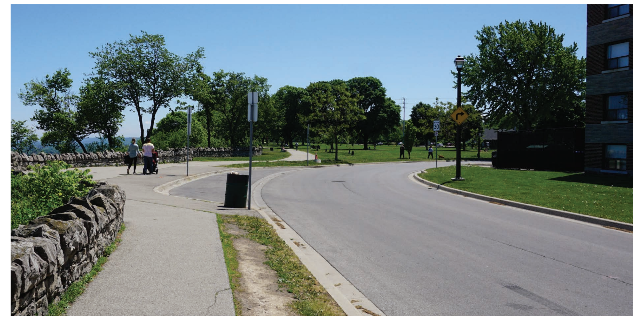
Existing Streetscape Conditions
