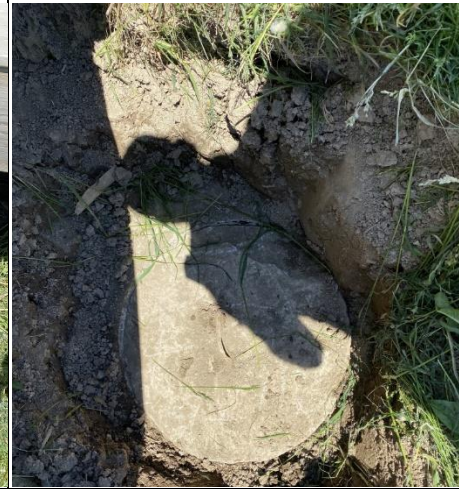
2. Septic tank discharge lid
