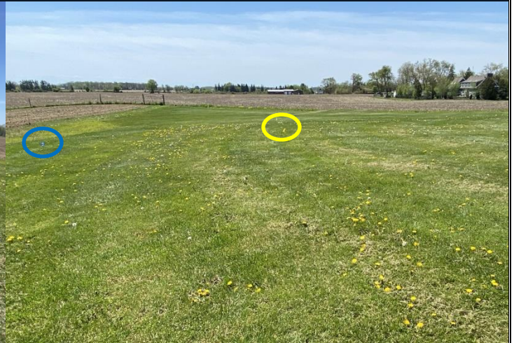
8. End of leaching field distribution lines – yellow flag represents end of lines (11.5m from property) blue flag is the 5m required setback
