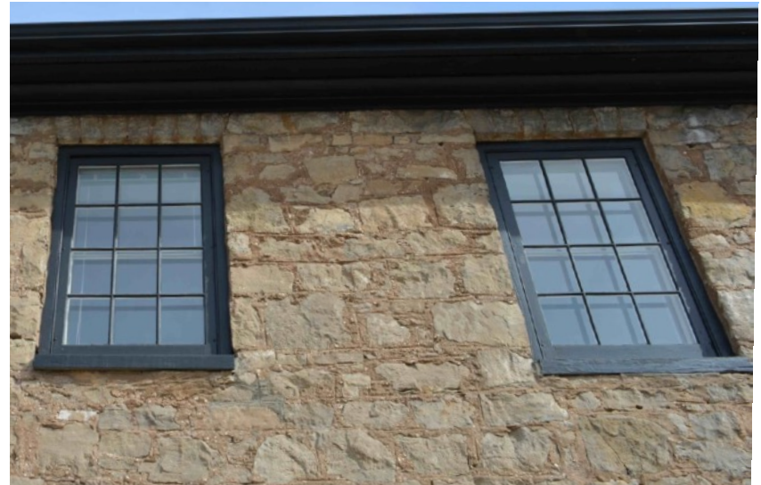
West elevation: window frames on 2nd storey appear to be in good repair upon visual review..
