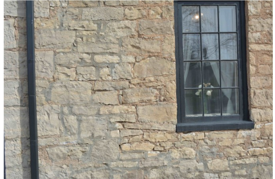
West elevation: ground level showing cementitious parging applied at the northern edge of the building.
