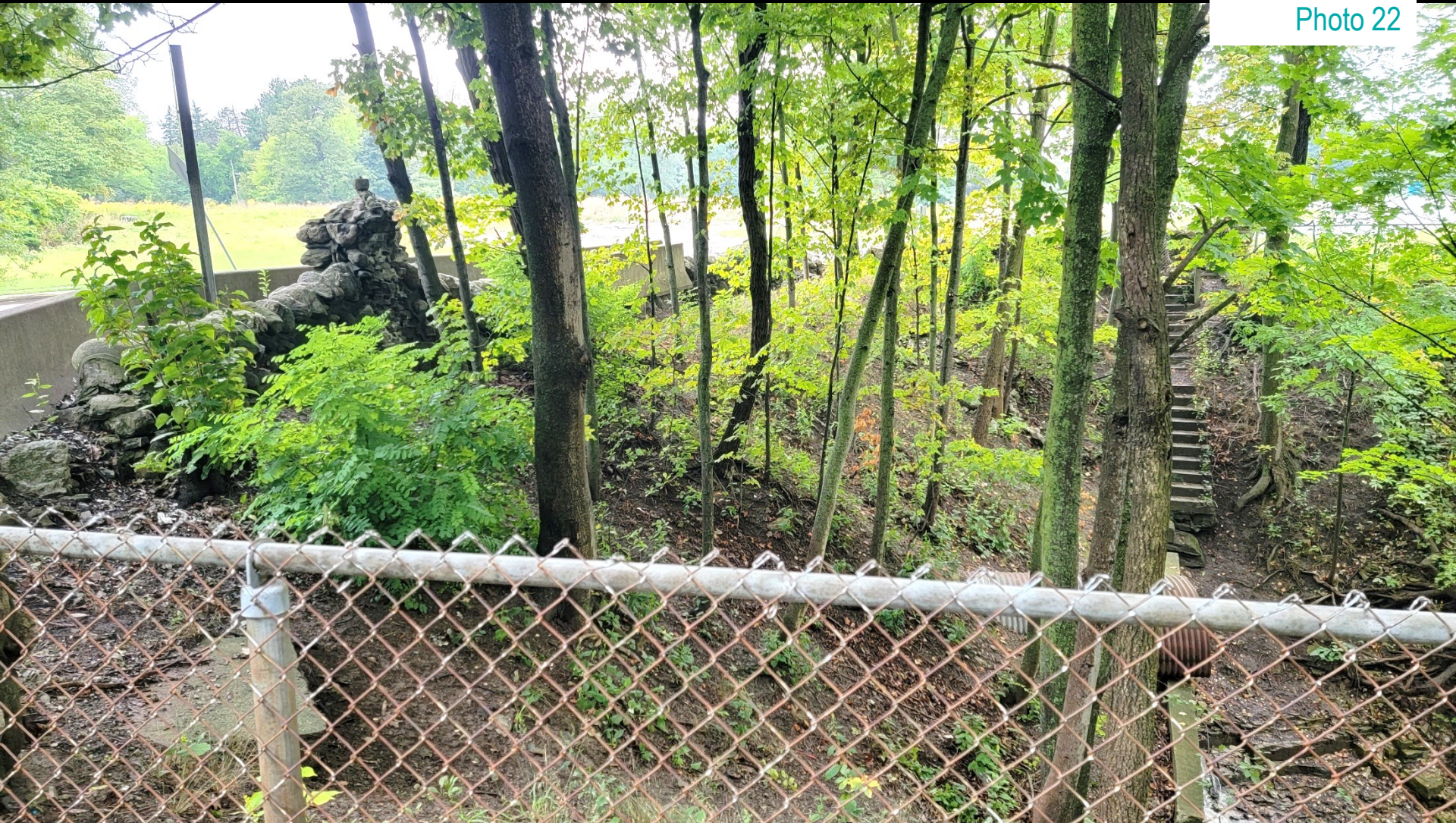
Stone wall and Escarpment stairs over Upper Sanatorium Falls
