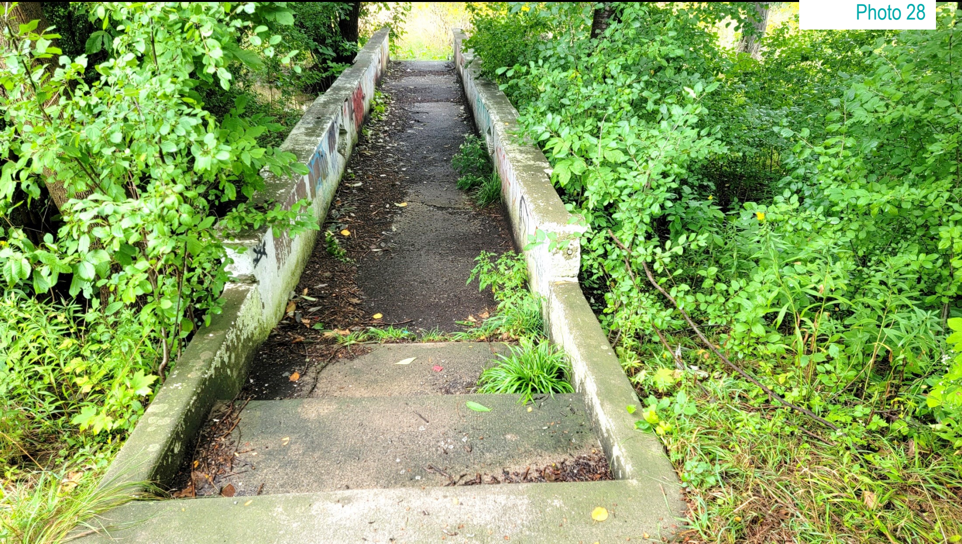
Pedestrian Bridge over the Tributary of Chedoke Creek
