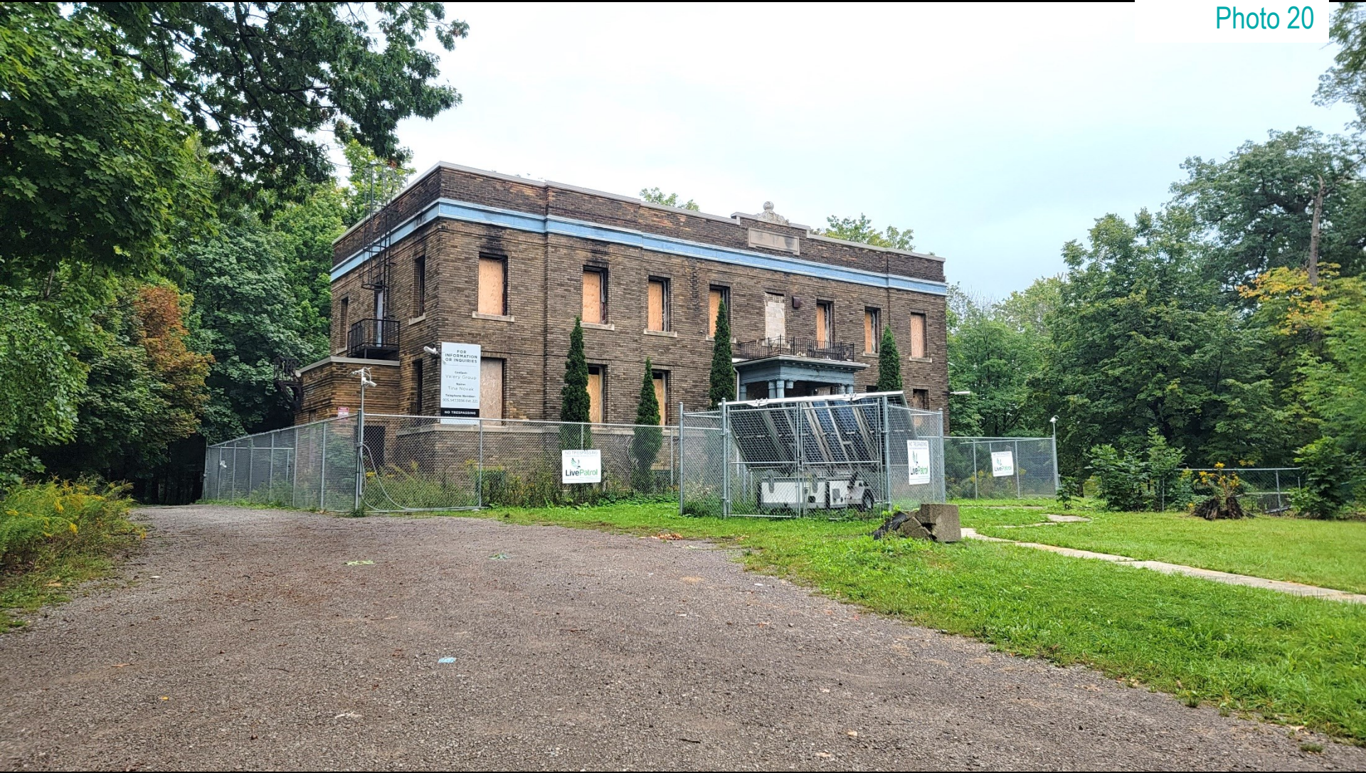
Long and Bisby Building (northwest corner)
