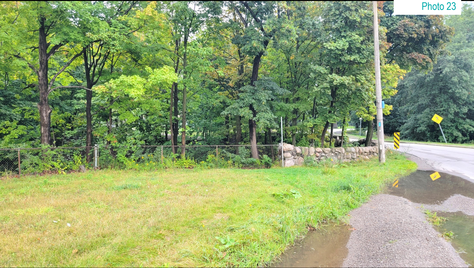
Stone wall over Upper Sanatorium Falls
