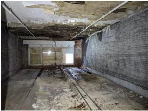
Fig 15: 24 King, 3<sup>rd</sup> floor level, severe water damage.
