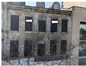
Fig 6: 18-20, upper façade, efflorescence noted
