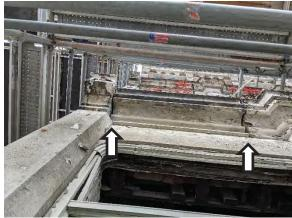
Fig 18: 28 King, E-most pier/spandrel, looking up note gaps in head joints.
