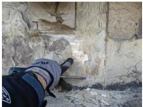
Fig 14: Subflorescence and stone flaking
