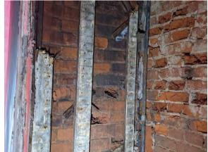
Fig 16: 24 King, saturated, deteriorated brick.
