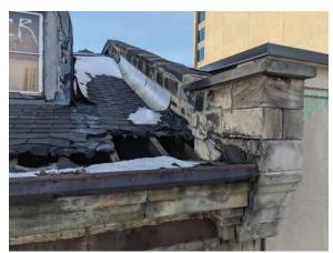
Fig 4: 18-20. Failed roof, pier at upper corner of façade
