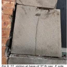
Fig 8: 22, cornice and bands of stone below. Sliding indicated. Fig 9: 22, sliding at base of 3rd flr pier, E side.
