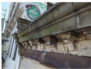
Fig 13: Deteriorated stone below cornice.
