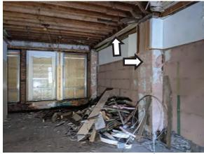
Fig 10: 22, beam and piers underside 3rd floor framing
