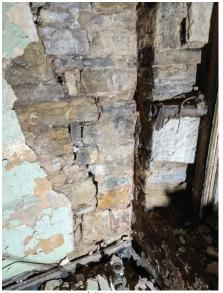
Fig 2: 18-20, 2nd floor, West return wall separation
