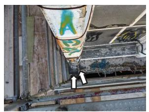
Fig 17: 28 King, E-most pier, looking down, note rotation, and gaps
