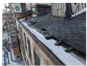
Fig 3: 18-20, failed roof rotted framing above cornice
