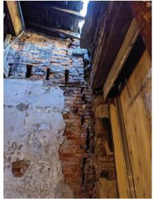
Fig 1: 18-20, 3<sup>rd</sup> floor, West return wall separation
