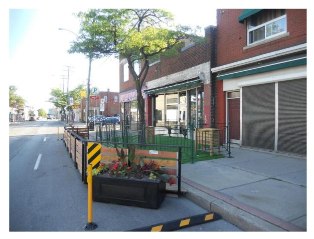
Image of a Pedestrian By-Pass Structure at The Argyle on Ottawa Street. The Patio area is on the sidewalk with the pedestrian by-pass structure in the parking space diverting traffic flow around the patio. The safety measures: Temporary Knock Down Bollard, Rubber Parking Stop Block, Yellow **Delineator and Planter** are shown.
