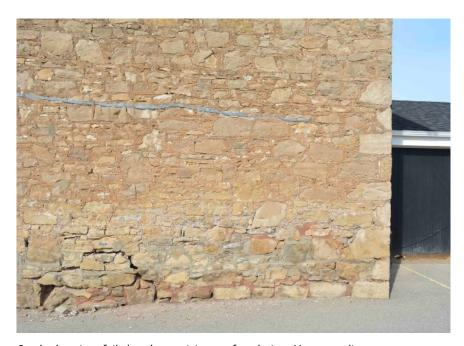
South elevation: failed and open joints at foundation. Movement lines are present at the midsection of this elevation.
