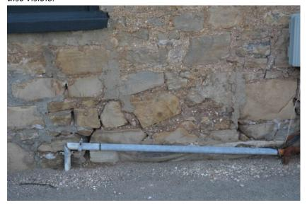
North elevation: failed and open joints, oxidization and metal anchors near foundation.
