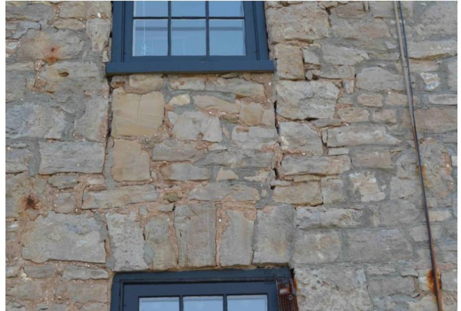
*West elevation: Recent repair and pointing work, parging and entire sections of stone removed below the 2nd storey window.*
