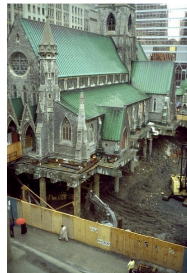
Caissons and pre-stressed beams support the Cathedral
