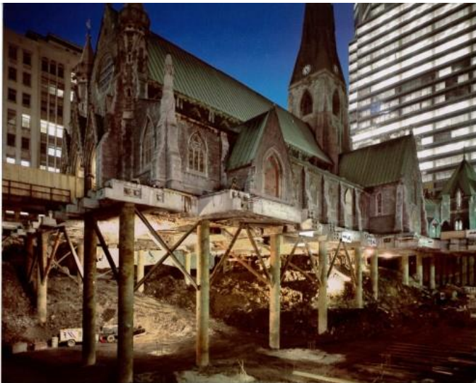
Caissons and pre-stressed beams support the Cathedral
