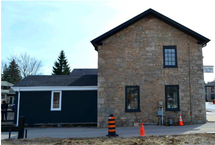
Marr House, 2021 (GBCA). North Elevation. Top left window opening closed in.
