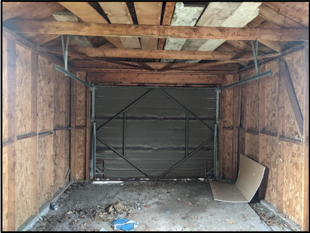
Interior of Garage, 19 Mill Street South, Waterdown City of Hamilton 2021
