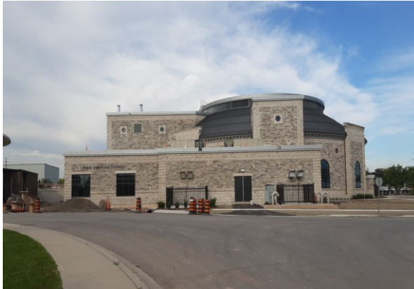
CONTRACT 1 Main Pumping Station
