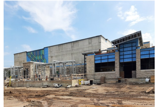
CONTRACT 3 Tertiary Treatment Upgrades
