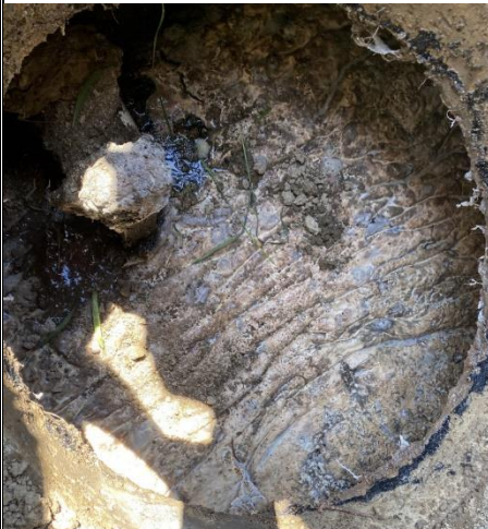
3. Condition of discharge portion of septic tank
