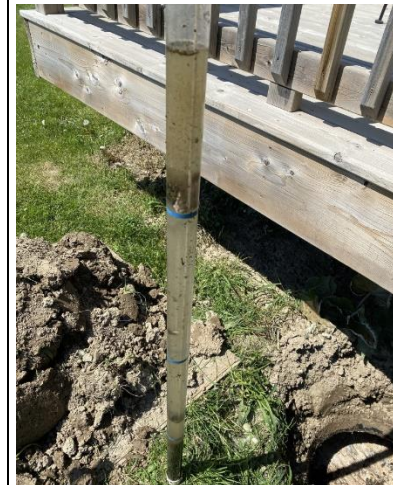
6. Sludge measurement of system (1 compartment) 35% solids – requires pump-out
