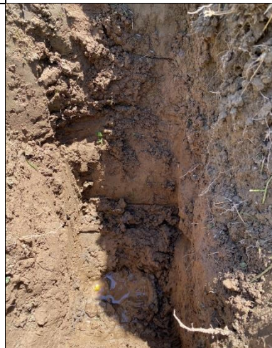
12. Soil profile of existing leaching field
