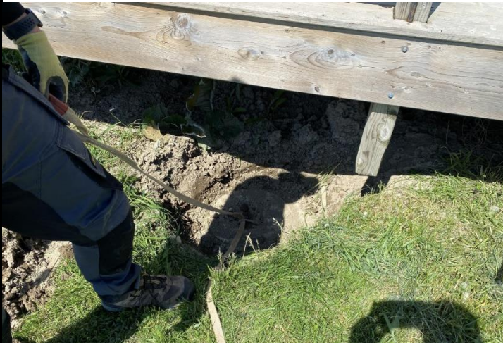
1. Location of Septic tank (inlet below deck)
