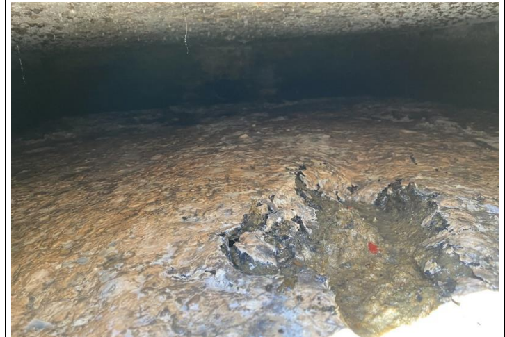
4. Interior condition of septic tank
