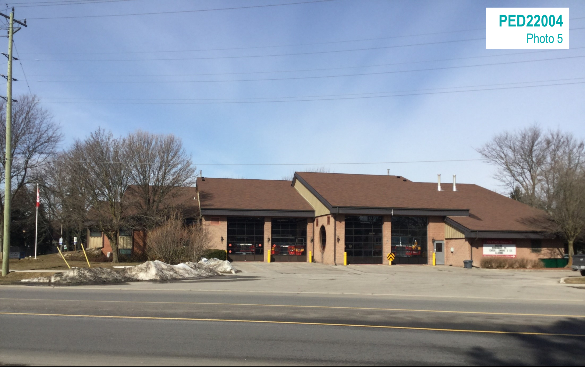
Photo of the fire hall at 365 Wilson Street West located across the street from the subject property to the north, as seen from Wilson Street West looking north
