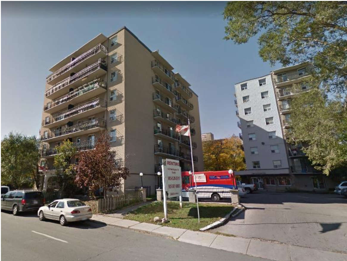
Figure 4 – Existing Rental Buildings to South of Subject Property
