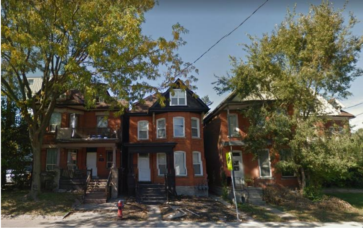
Figure 5 – Existing Single Detached Residential Dwellings to North of Subject Property
