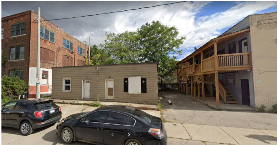
Figure 5 – Semi-Detached Dwelling at 6 – 8 Steven St and Rear of 571 – 575 King St E (from Steven Street)
