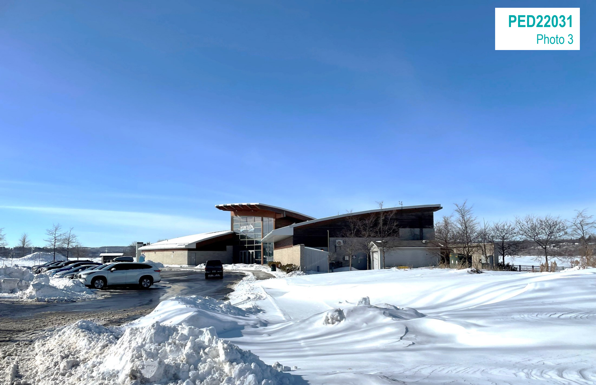
View of adjacent lands to the northwest
