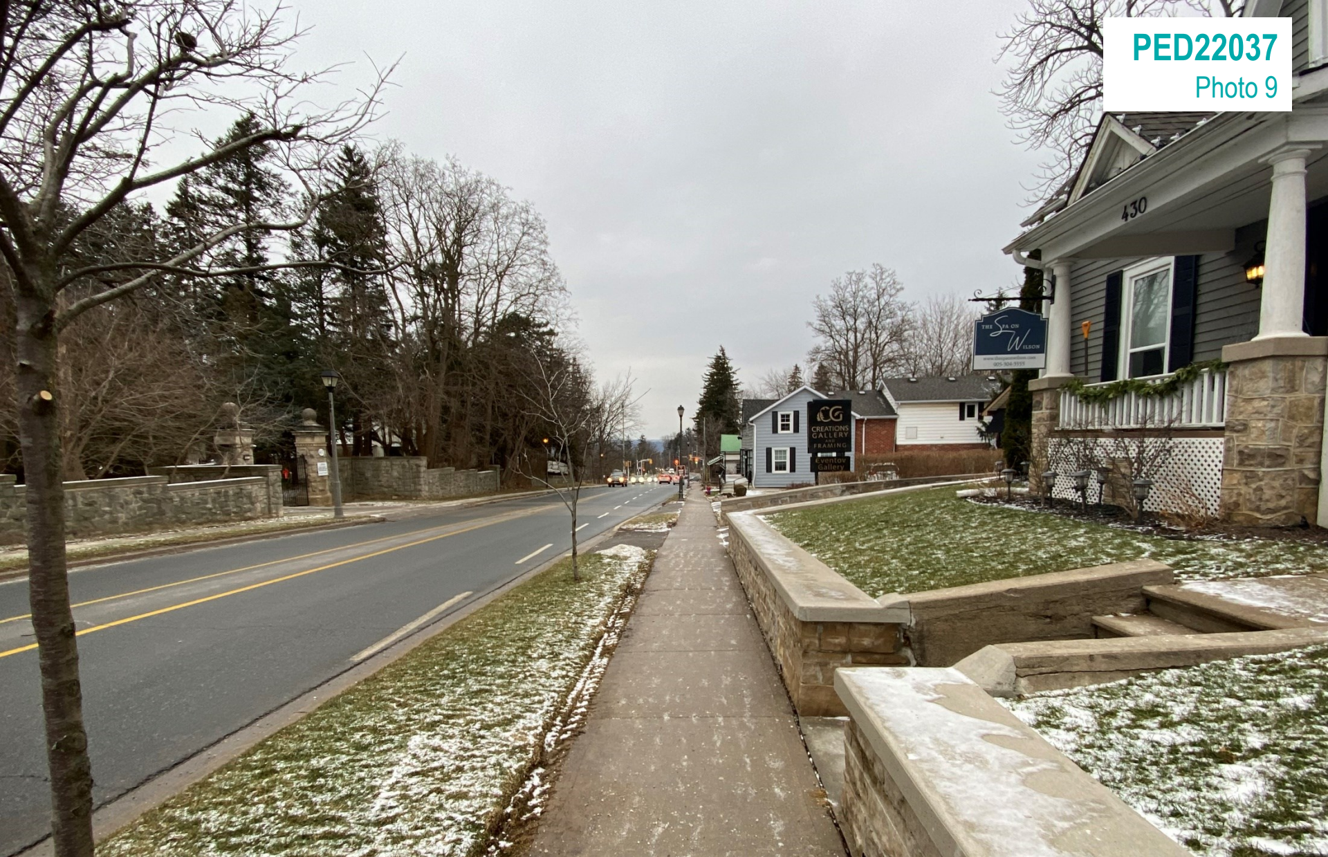
View looking north on Wilson Street East
