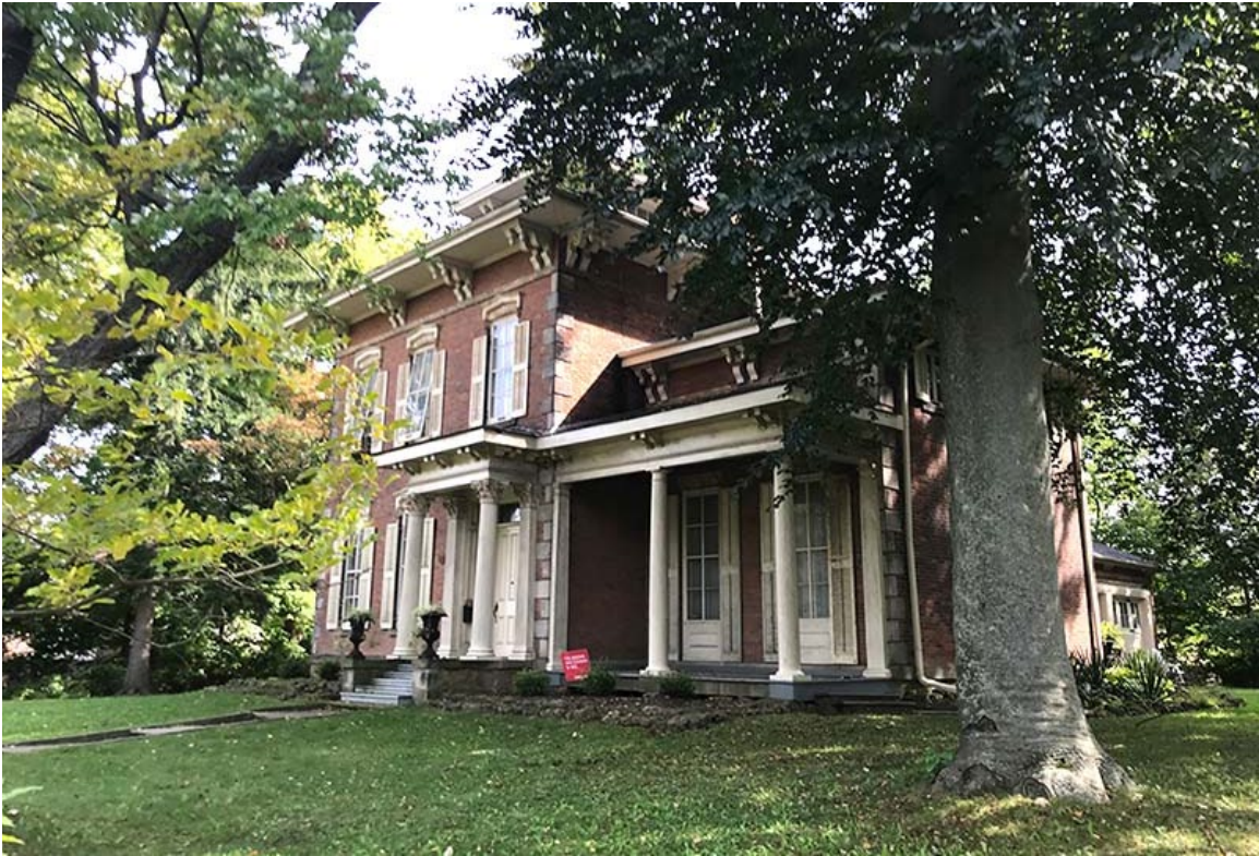
“Balindalloch” at 192 Governor’s Road: a notable example of the Italianate style, featuring a hipped roof with very wide eaves, elaborate paired wood brackets, stone corner quoins and a front porch with Corinthian columns and an entablature supporting a roof with wide eaves featuring smaller paired
