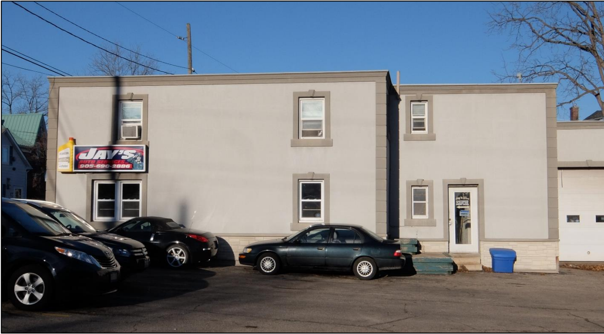
Image 5: 19 Flamboro Street side (south) facade clad in stucco, December 2021 (City of Hamilton)
