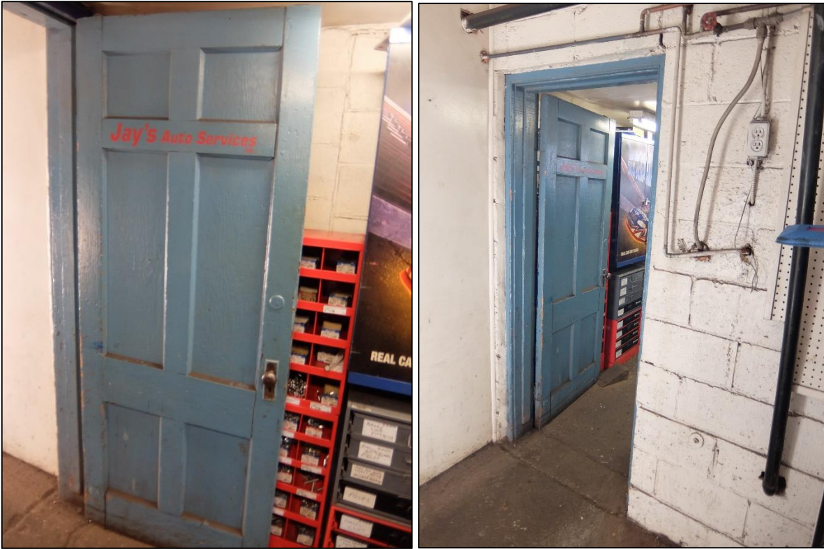
Images 17 and 18: Remaining interior six-panel wood door located in the entrance to the first interior garage, December 2021 (City of Hamilton)
