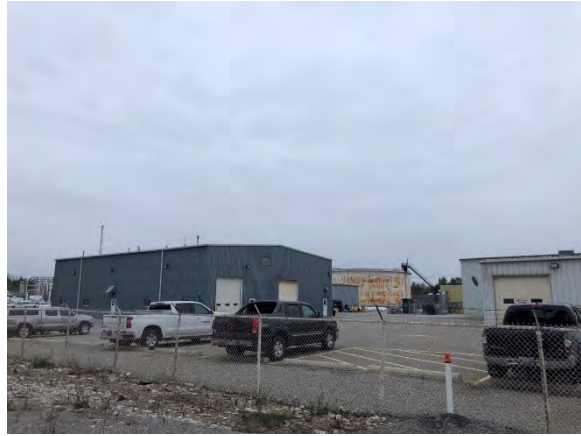
Photo 10: View of existing disturbance (facility), facing northeast
