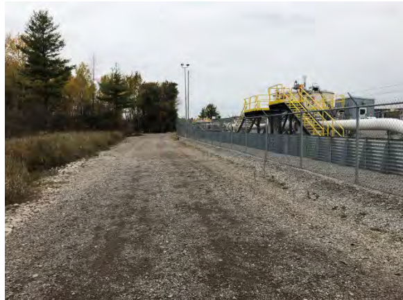
Photo 8: View of existing disturbance (access road and facility), facing north
