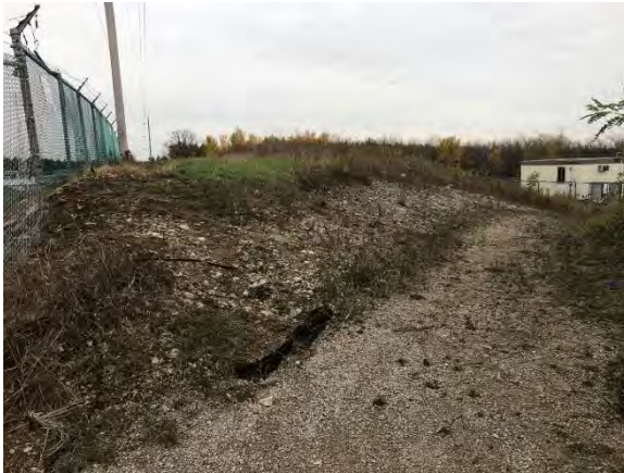
Photo 1: View of existing disturbance (artificial berm), facing southwest
