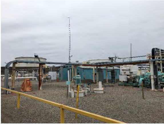
Photo 9: View of existing disturbance (facility), facing northeast
