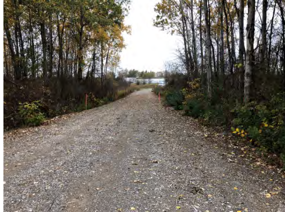
Photo 6: View of existing disturbance (access road), facing northwest
