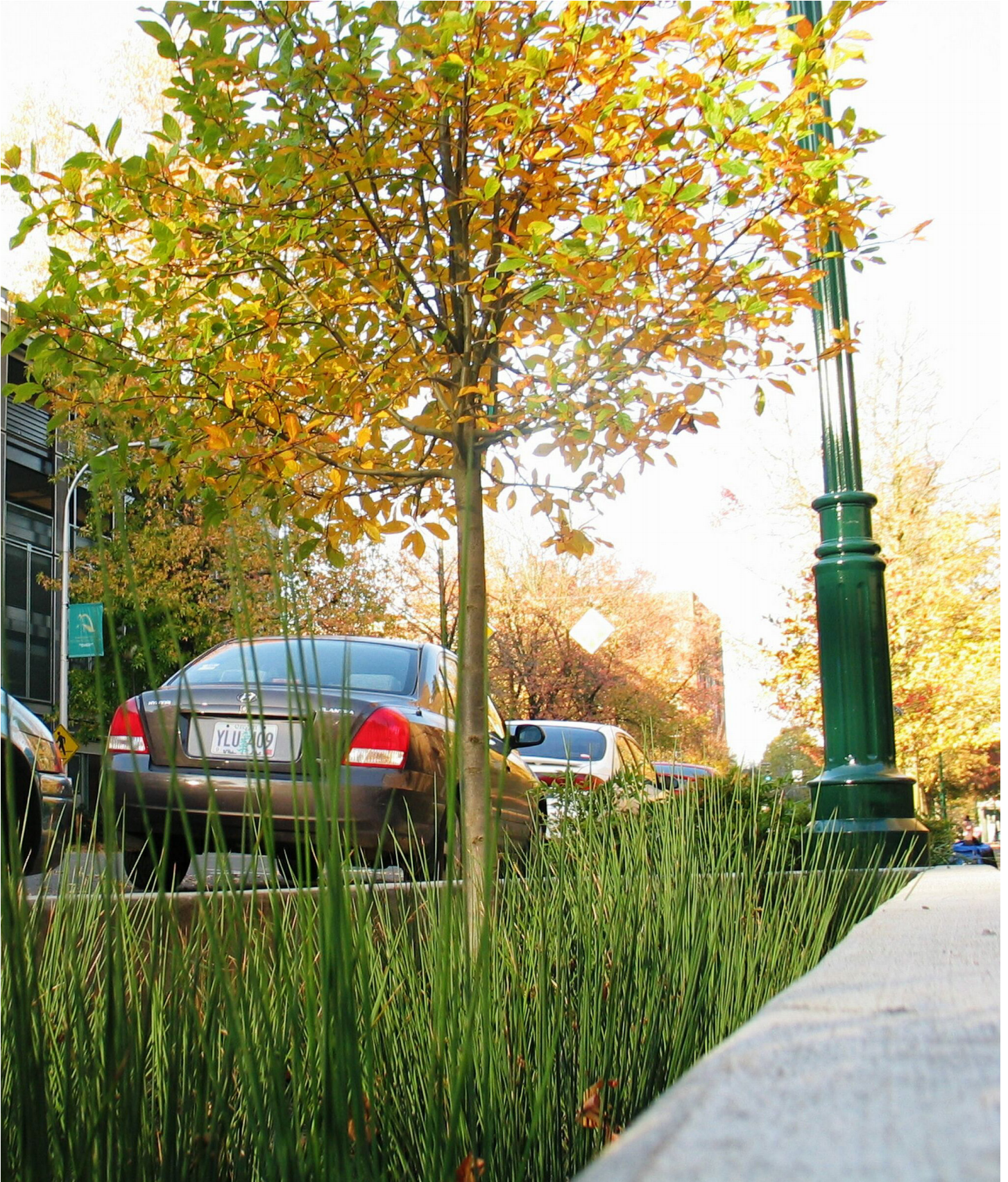
Example of biofiltration trench within the public boulevard to increase soil infiltration and improve stormwater management (Brook McIlroy).
