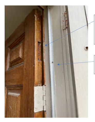
At some point the hinge position has been changed. Wood is rotten and will not hold a screw. New location below tenon is weak. Propose new 1 ½ pr hinges in lieu of 1 pr existing.
