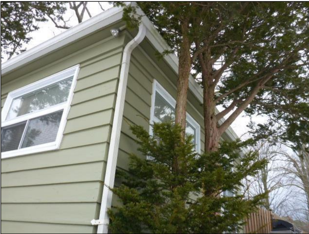
Image 4: Typical exterior siding and windows
