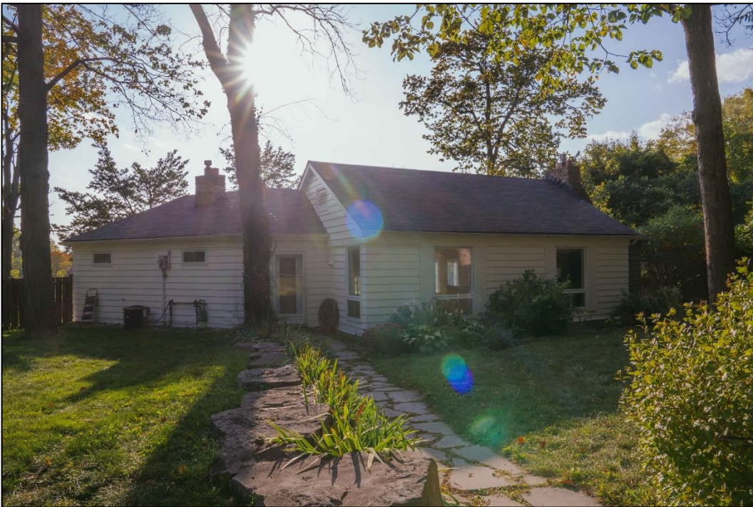
Image 2: Front façade, close-up
