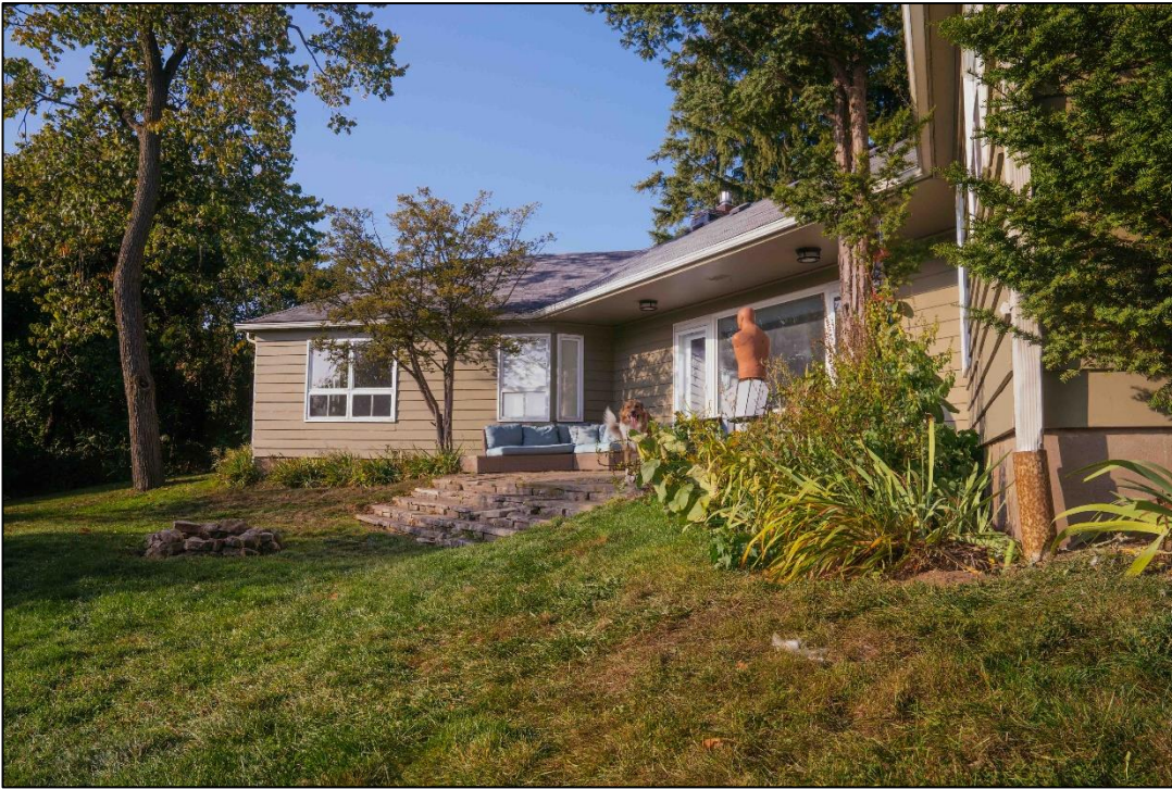
Image 3: Rear (west) exterior facades
