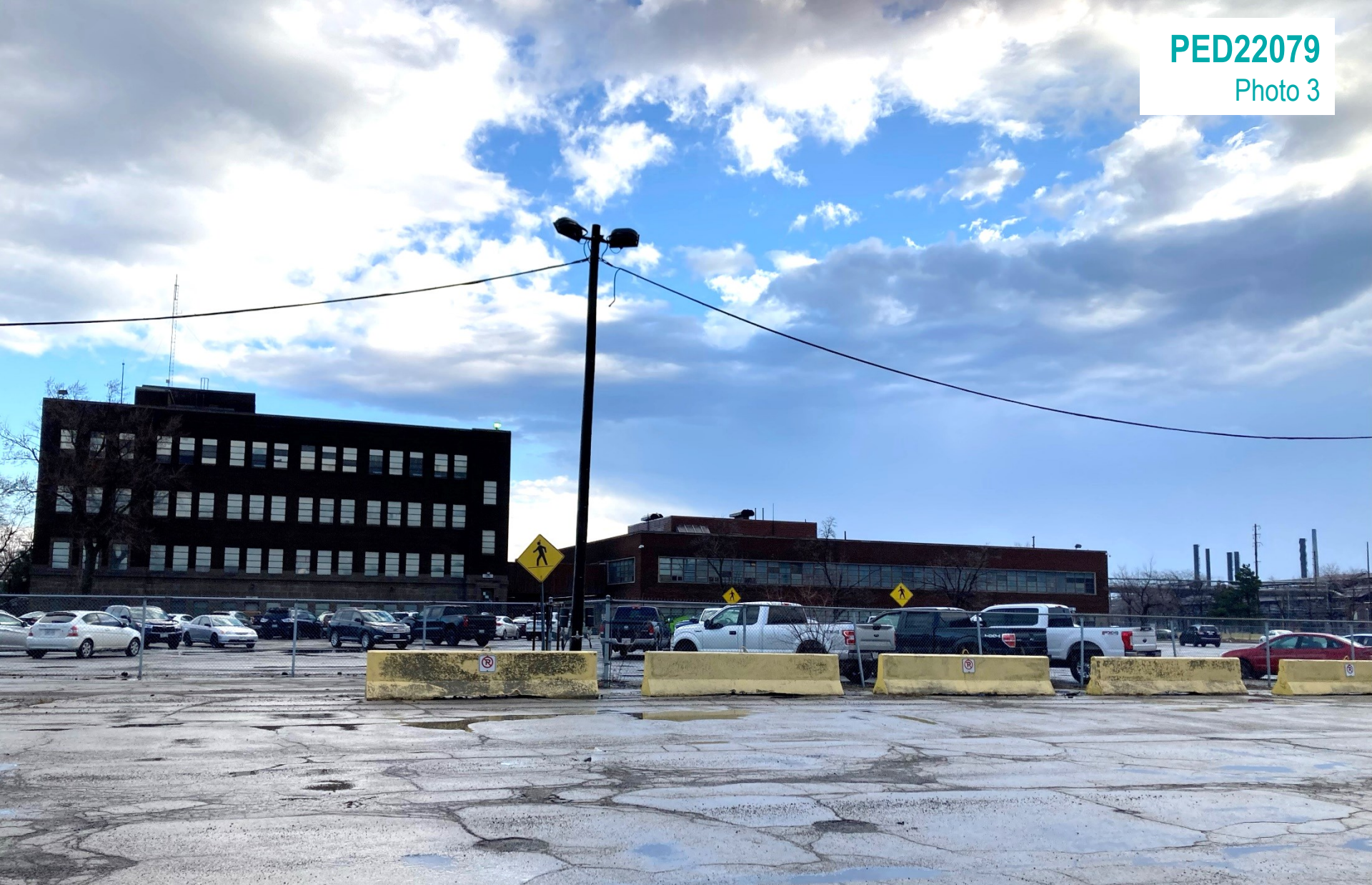
Looking north towards the Industrial lands
