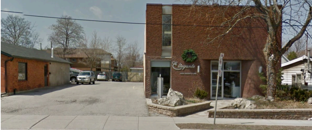
Figure 5: 528 Upper James Street, Abutting Commercial Property (South) (Google Maps)
