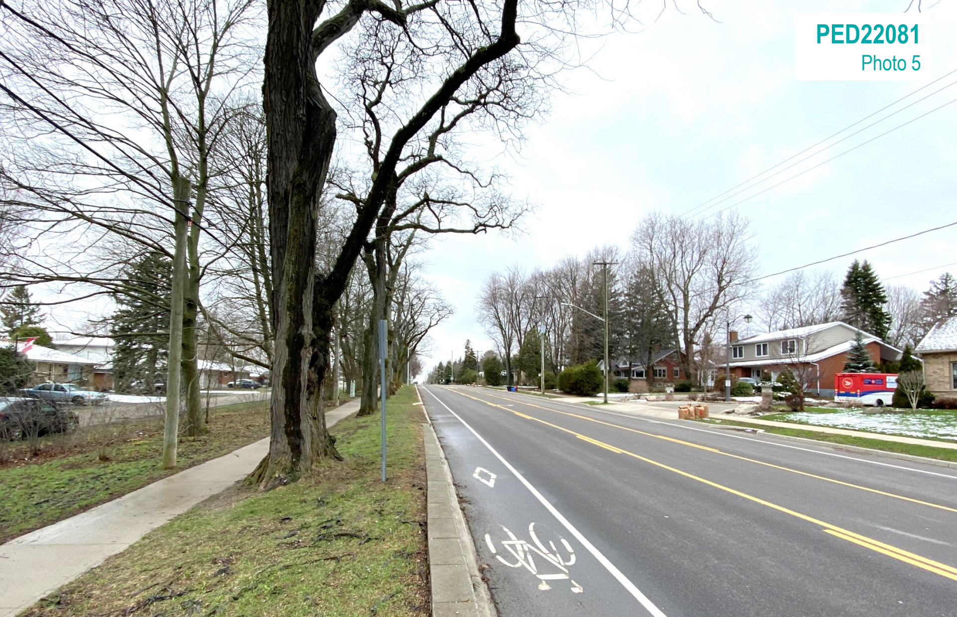
View looking south west on Wilson Street West
