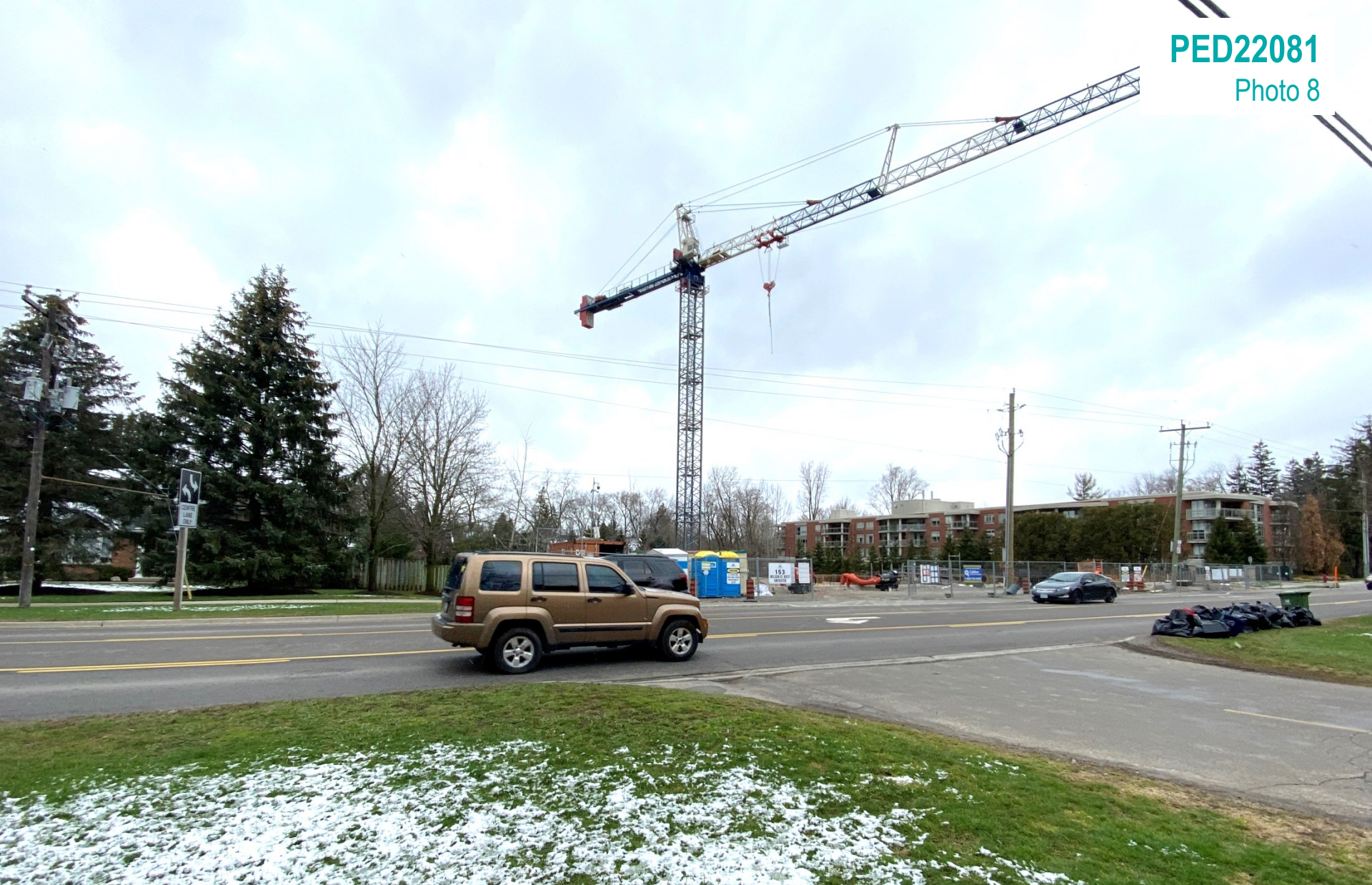
Building under construction at 153 Wilson Street West
