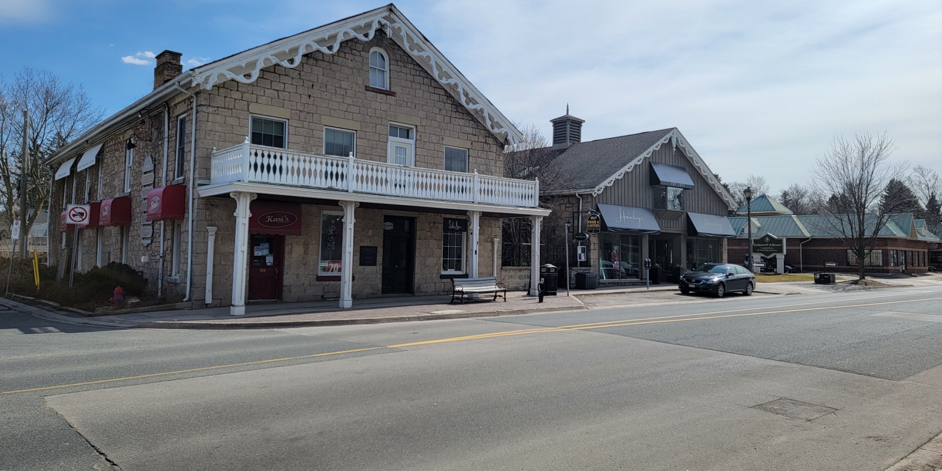
South of subject site along east side of Wilson Street East
