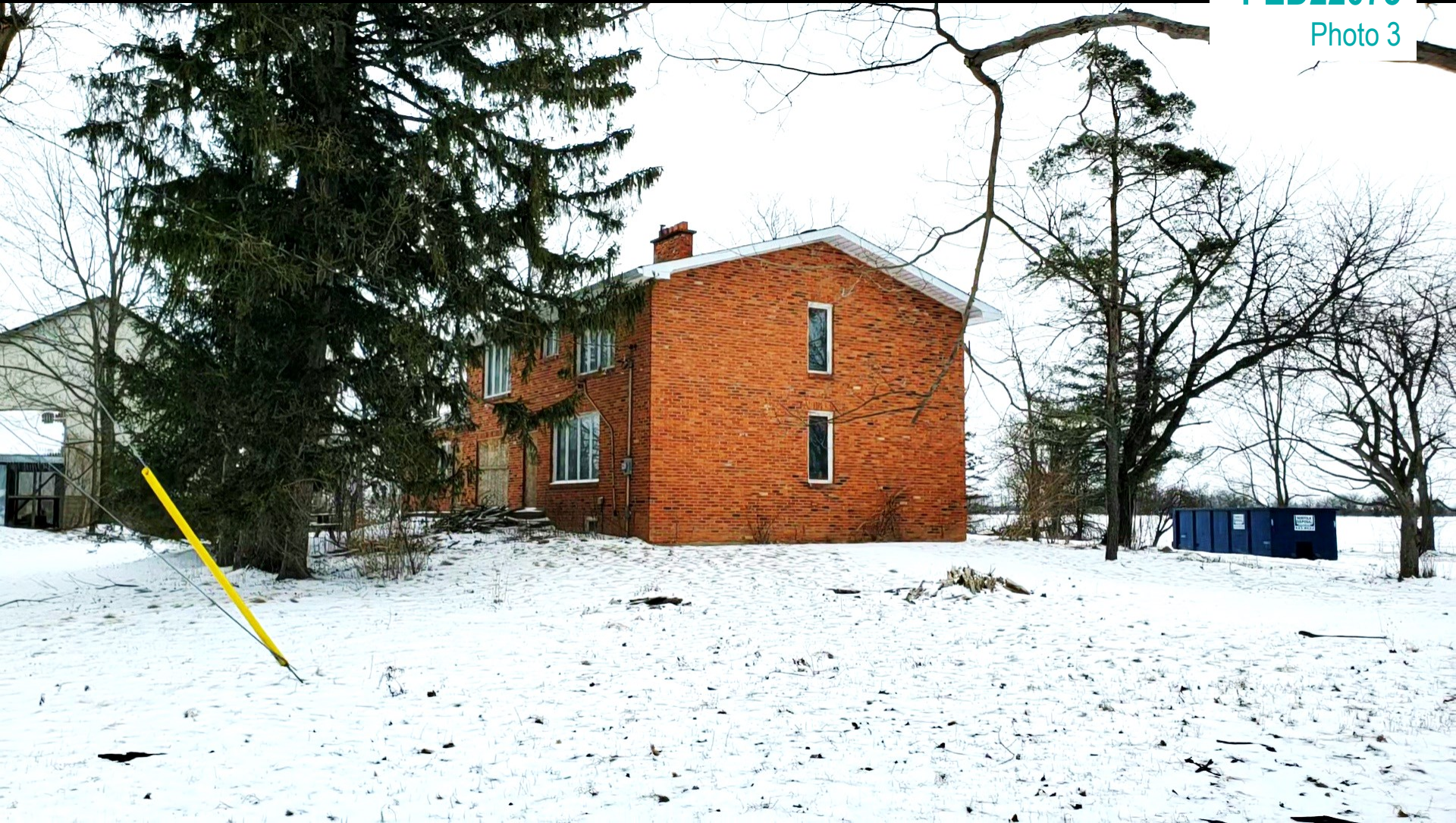
View from the central portion of the subject from the Haldibrook Road looking northwest
