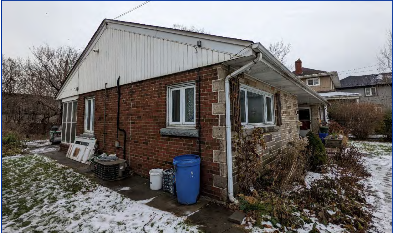
Figure 12: View of the south elevation of the residence
