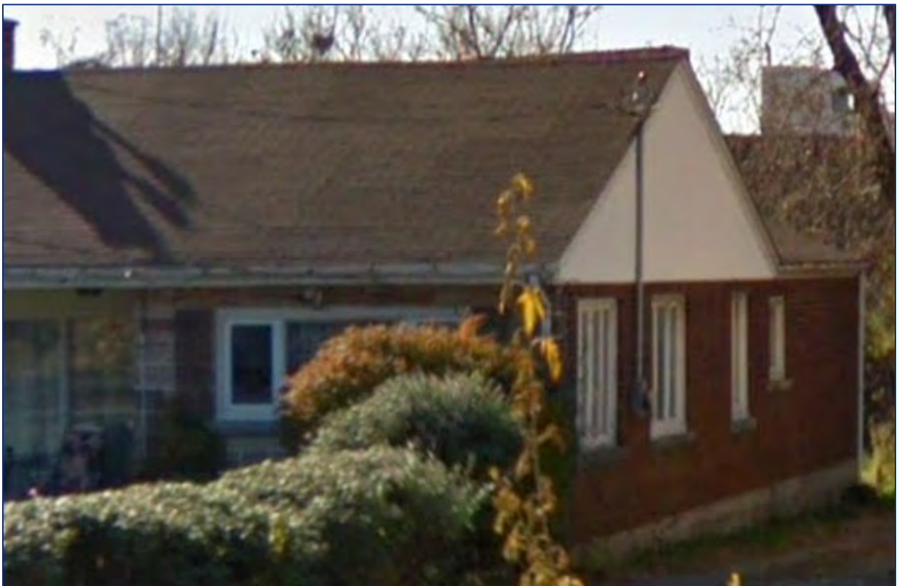
Figure 15: View of the north elevation of the residence and its rear addition; Source: Google Streetview November 2016
