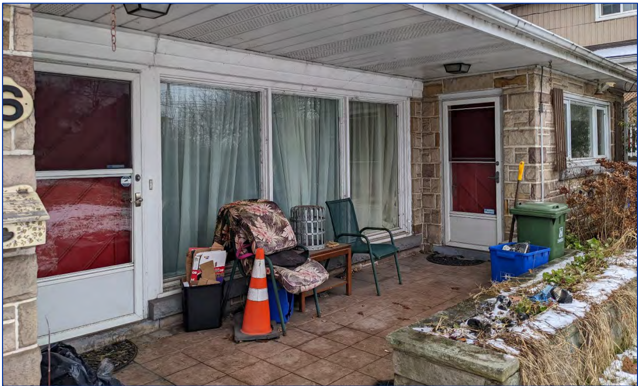
Figure 19: View of the inset covered porch
