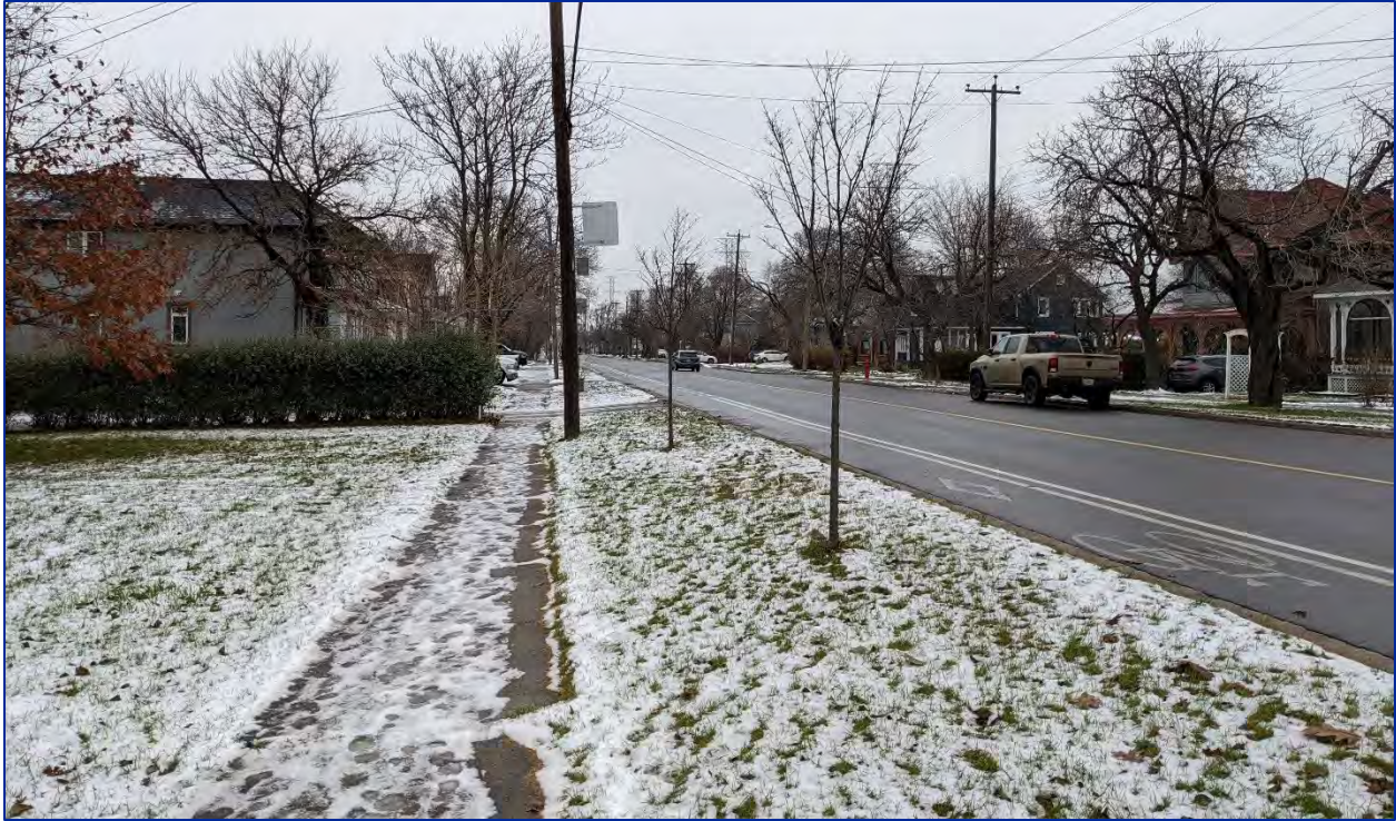
Figure 26: View north along Beach Boulevard from the sidewalk in front of the Property
