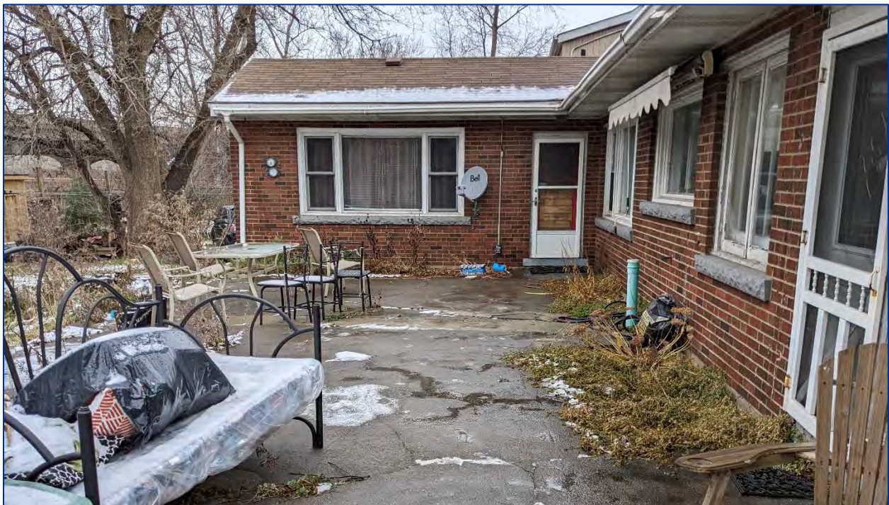
Figure 13: View of the south elevation of the rear addition
