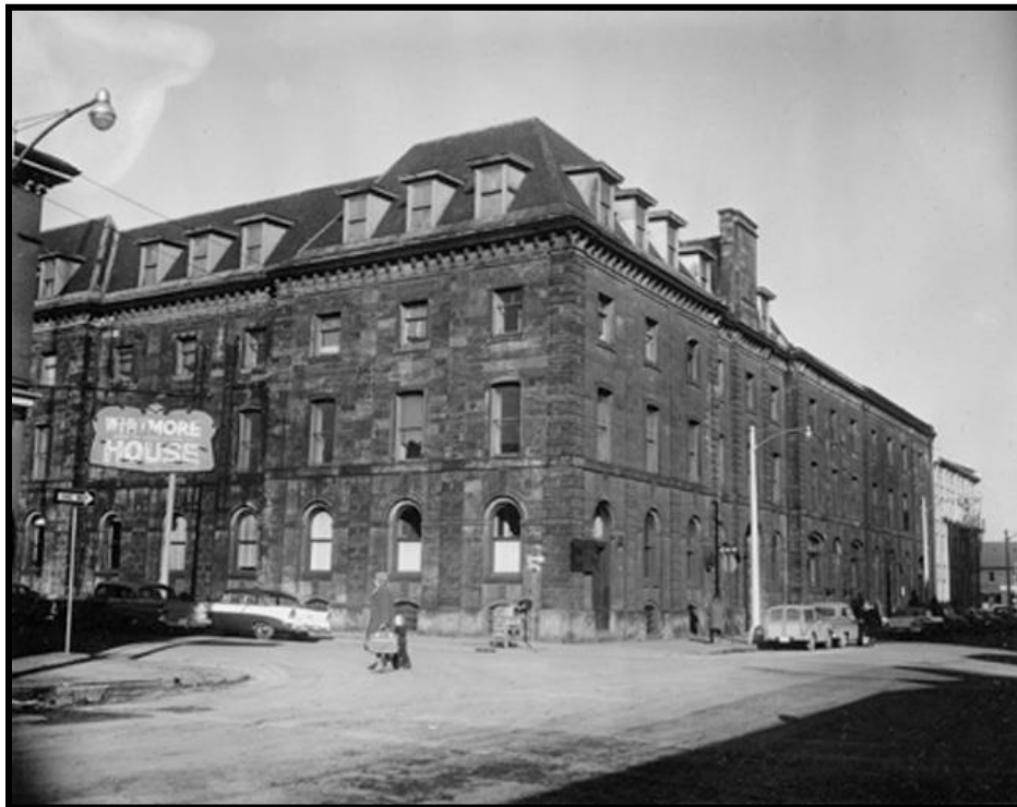
Plate 12: Stone Building at 56 York Boulevard (HPL LHA no date)
