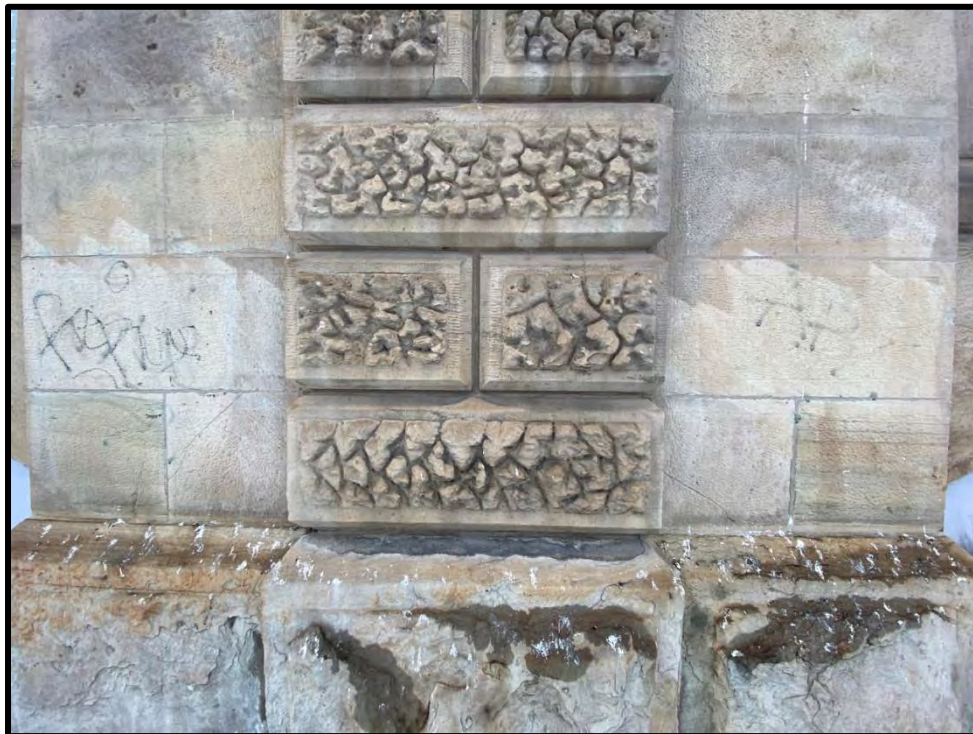
Image 10: Vermiculated Stone Pilaster and Dressed Stone – Detail (Photo taken on December 8, 2021; Facing North)
