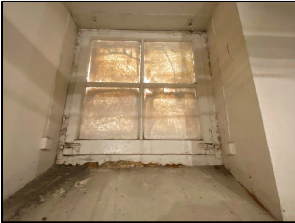
Image 183: Basement Brick Building – Window Detail (Photo taken on December 8, 2021; Facing East)
