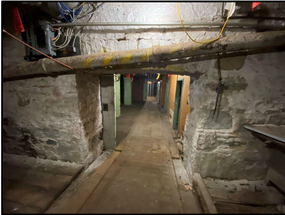
Image 151: Basement Stone Building – Interior (Photo taken on December 8, 2021)
