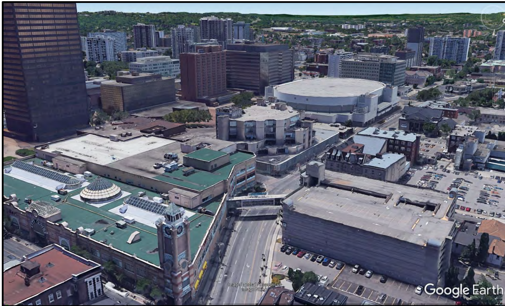
Figure 1: Oblique Image of Context (Current) (Google Earth 2022)
