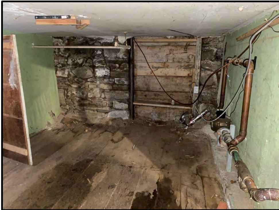
Image 153: Basement Stone Building – Interior (Photo taken on December 8, 2021)
