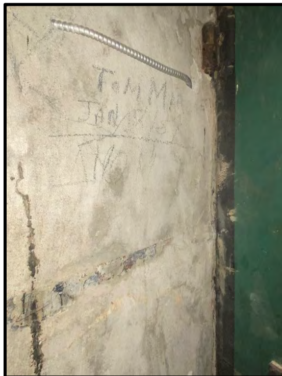
Image 156: Basement Stone Building – Vault Graffiti (Photo taken on December 8, 2021)
