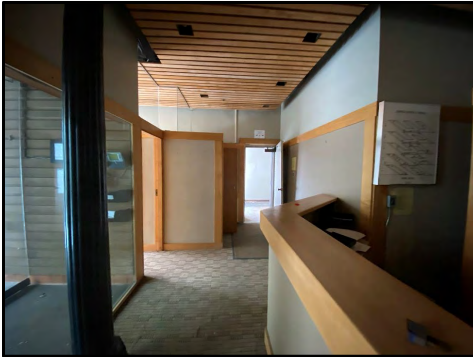
Image 57: First Floor – Interior (Photo taken on December 8, 2021; Facing West)
