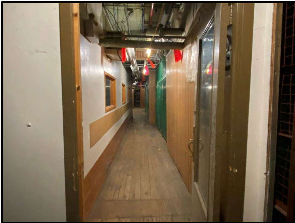
Image 144: Basement Stone Building – Interior (Photo taken on December 8, 2021)
