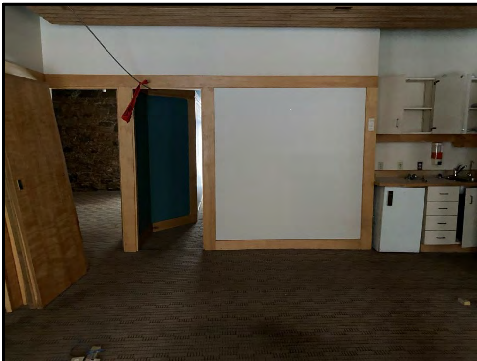
Image 72: First Floor – Interior (Photo taken on December 8, 2021; Facing West)
