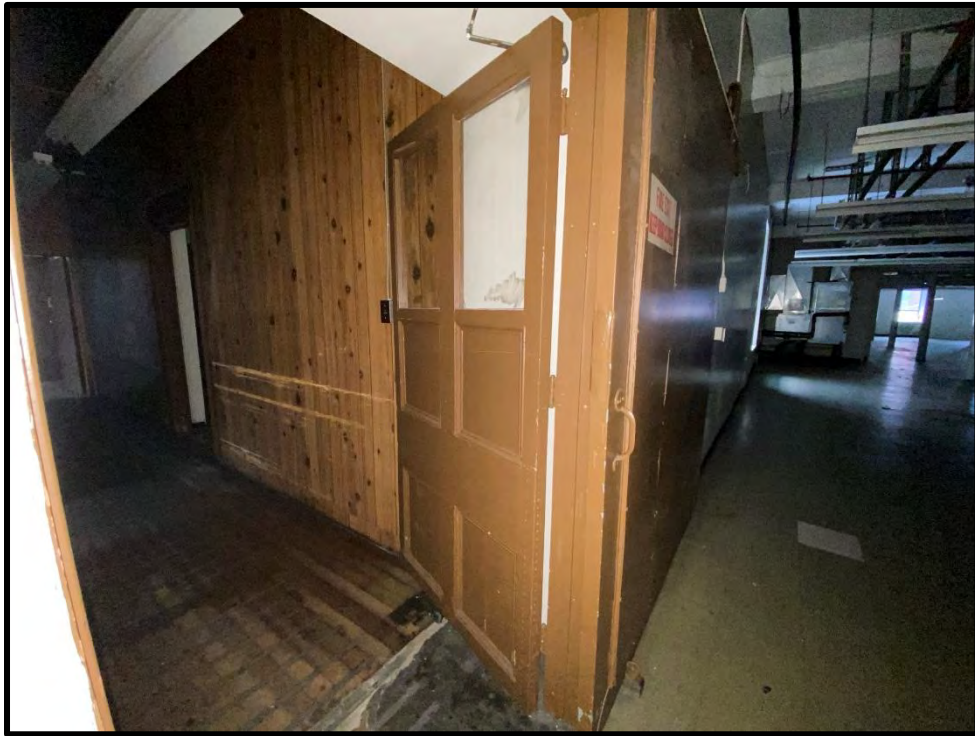
Image 117: Second Floor North Addition – Interior (Photo taken on December 8, 2021; Facing Northeast)
