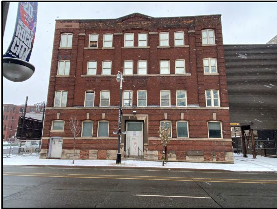
Image 37: York Street Front Façade (Photo taken on December 8, 2021; Facing North)
