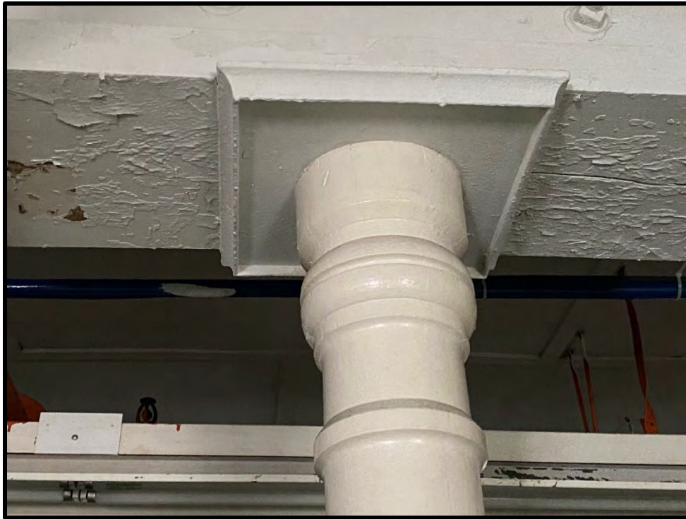
Image 127: Third Floor Stone Building – Support Pillar (Photo taken on December 8, 2021)
