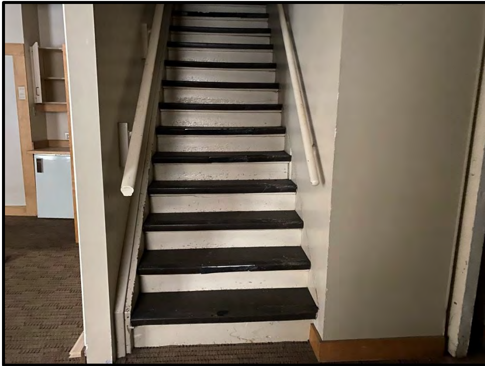
Image 75: First Floor Interior – Staircase Detail (Photo taken on December 8, 2021; Facing West)
