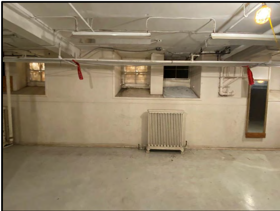
Image 182: Basement Brick Building – Interior (Photo taken on December 8, 2021; Facing East)
