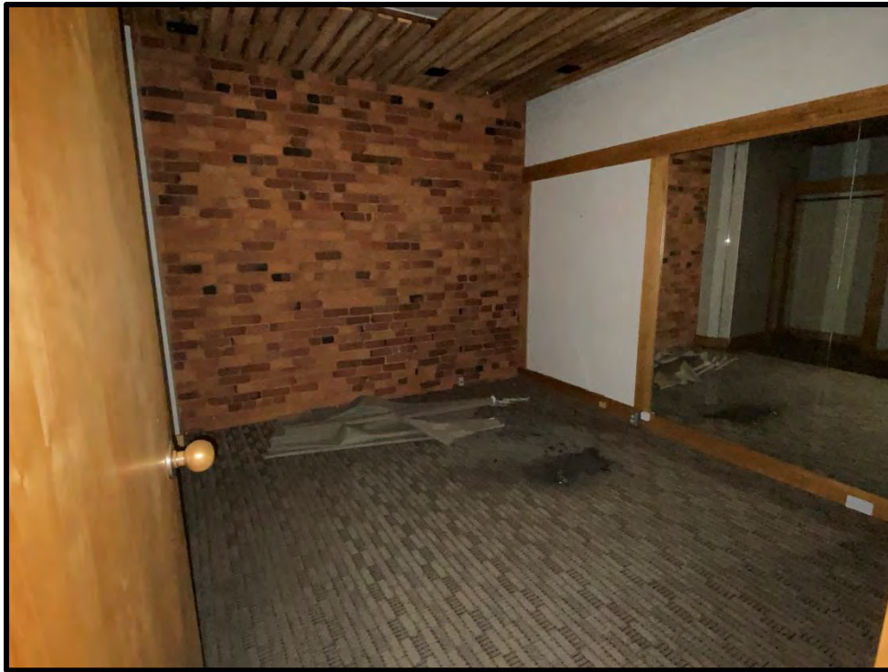
Image 71: First Floor – Interior (Photo taken on December 8, 2021; Facing Southwest)
