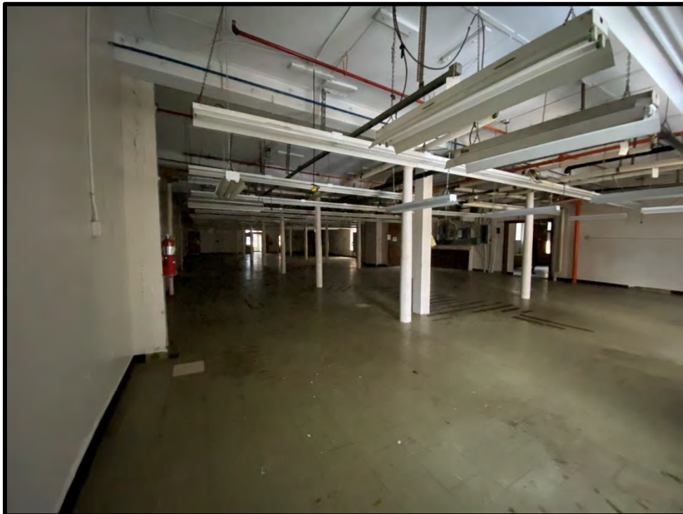
Image 114: Second Floor North Addition – Interior (Photo taken on December 8, 2021; Facing Southeast)
