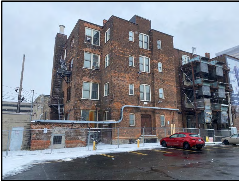
Image 45: West Elevation Showing Elevator Shaft (Photo taken on December 8, 2021; Facing Southeast)
