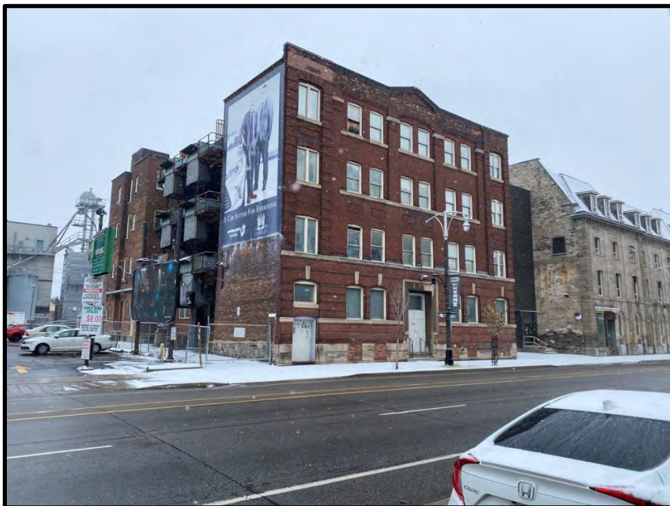
Image 42: South and West Elevations (Photo taken on December 8, 2021; Facing Northeast)
