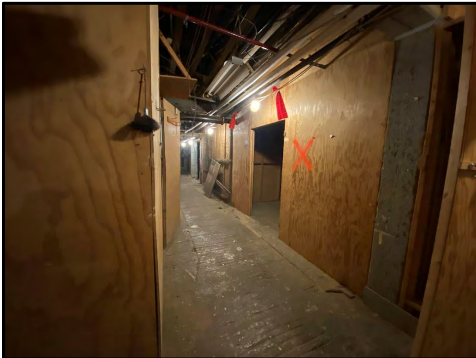
Image 152: Basement Stone Building – Interior (Photo taken on December 8, 2021)
