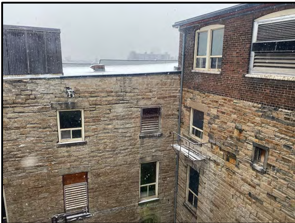
Image 34: Courtyard (Photo taken on December 8, 2021; Facing Northeast)
