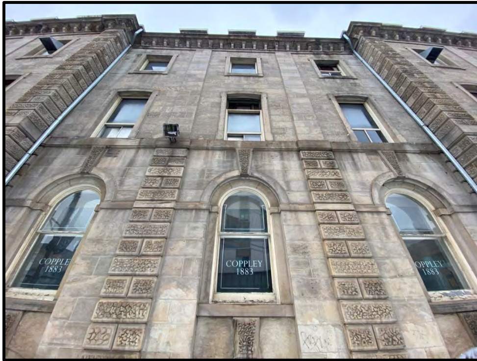
Image 9: Detail of Central Section of York Street Front Façade (Photo taken on December 8, 2021; Facing North)
