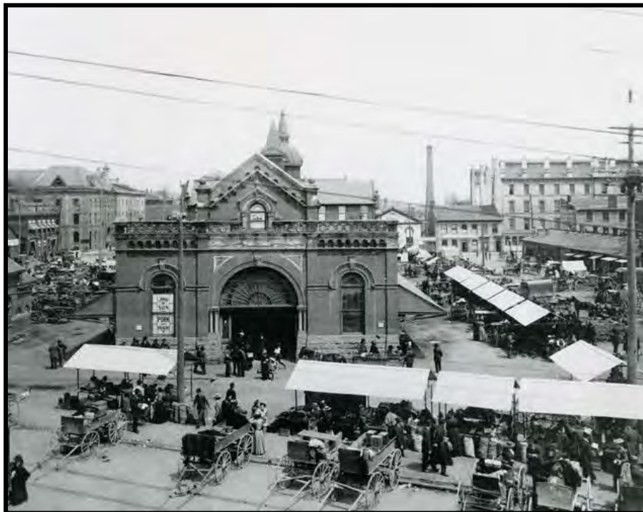
Plate 2: View of Hamilton Market with Stone Subject Building at Left (HPL LHA circa 1893)
