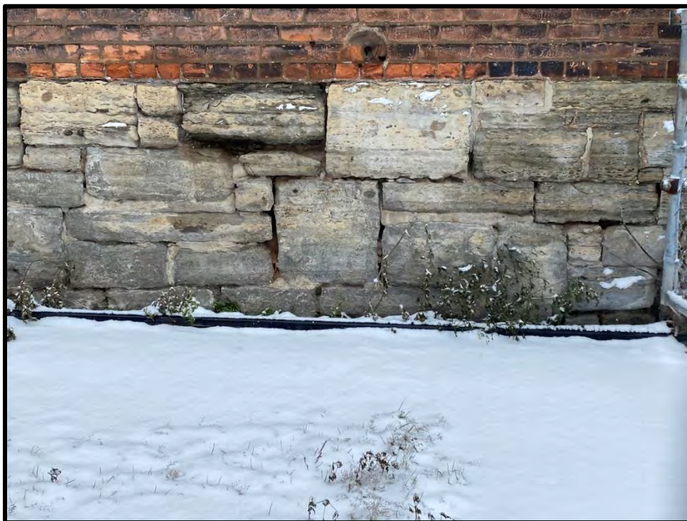
Image 44: Detail of Stone Foundation Brick Coursing on West Elevation (Photo taken on December 8, 2021; Facing East)
