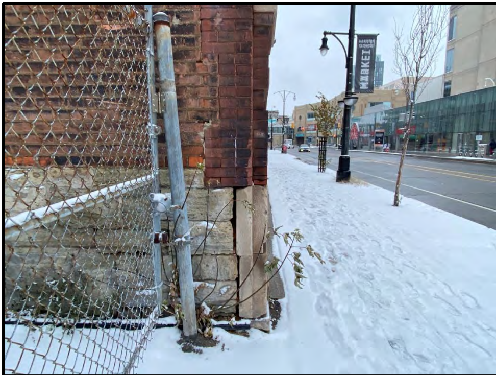
Image 38: Detail of Front Façade Cladding (Photo taken on December 8, 2021; Facing East)
