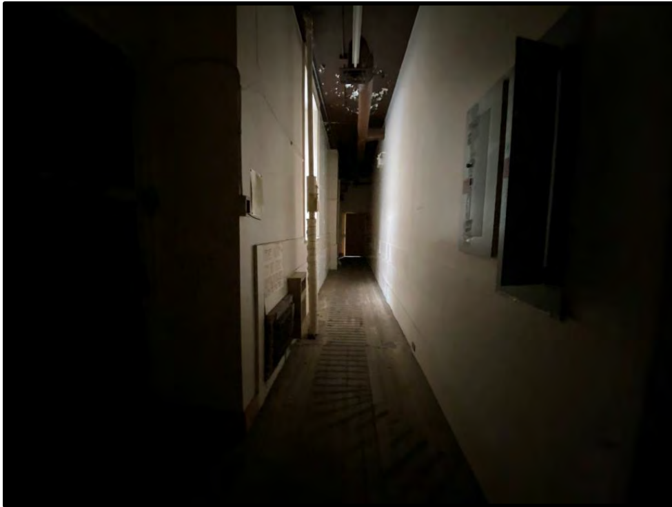
Image 89: First Floor North Addition – Interior (Measurements taken on December 8, 2021; Facing West)
