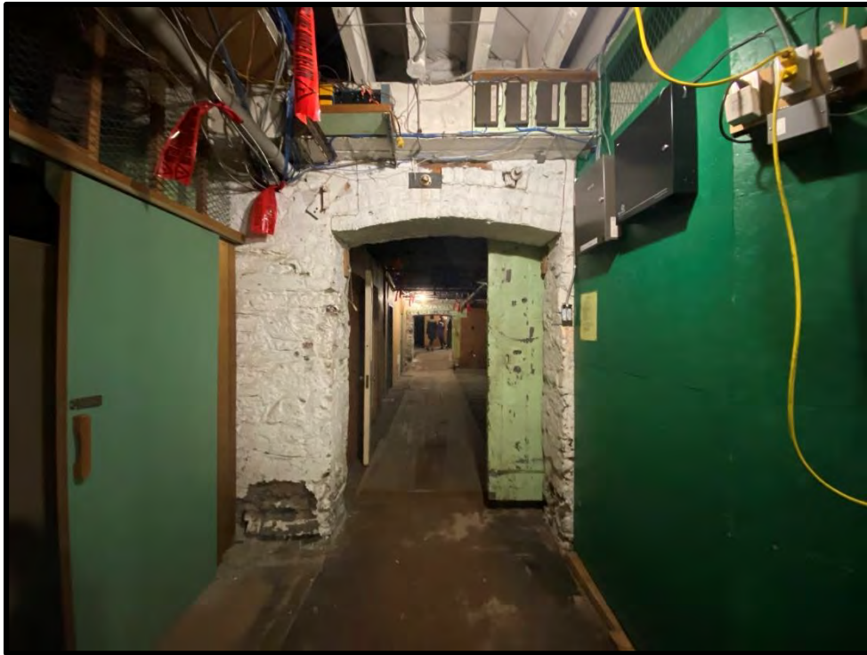
Image 149: Basement Stone Building – Interior (Photo taken on December 8, 2021)
