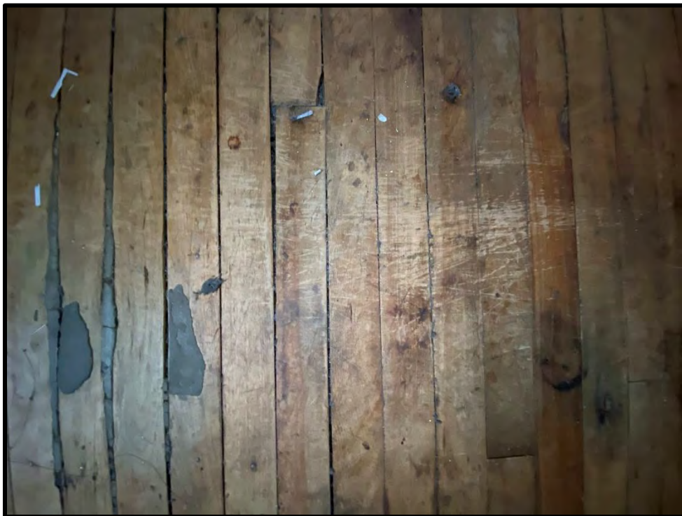
Image 132: Second Floor Hardwood Flooring – Detail (Photo taken on December 8, 2021)
