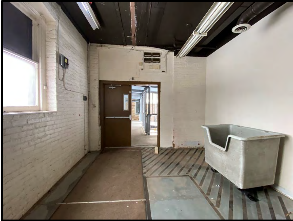
Image 167: First Floor Brick Building – Interior (Photo taken on December 8, 2021; Facing East)
