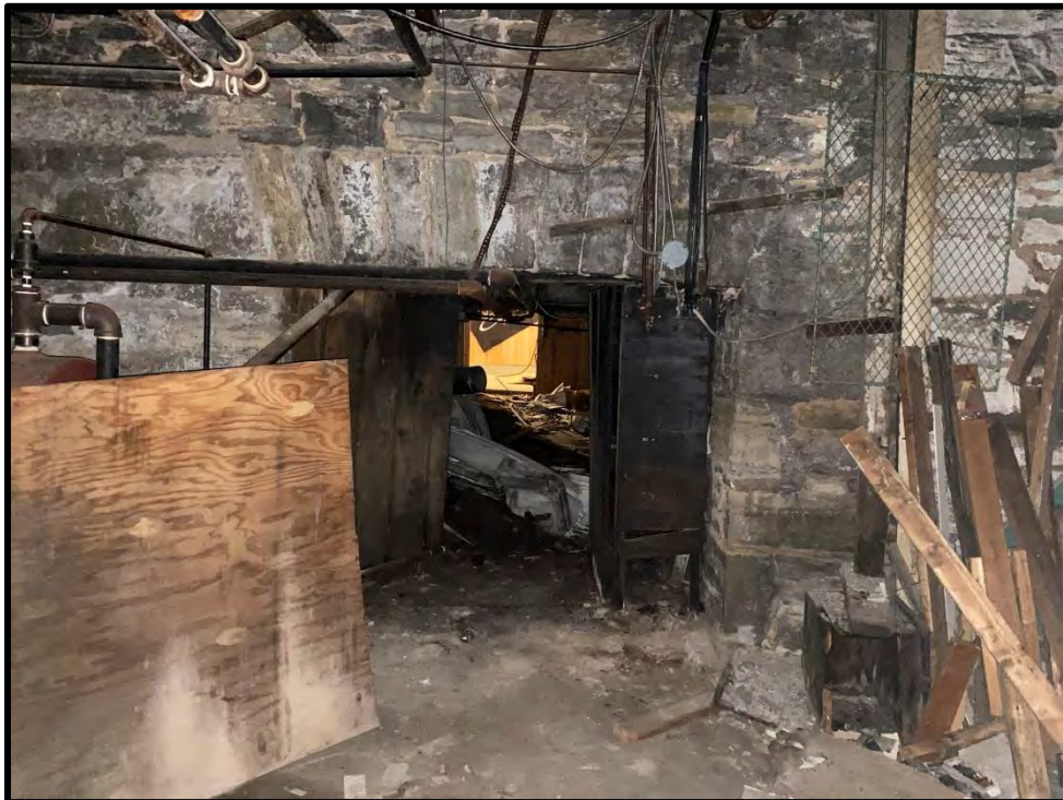
Image 146: Basement Stone Building – Interior (Photo taken on December 8, 2021)
