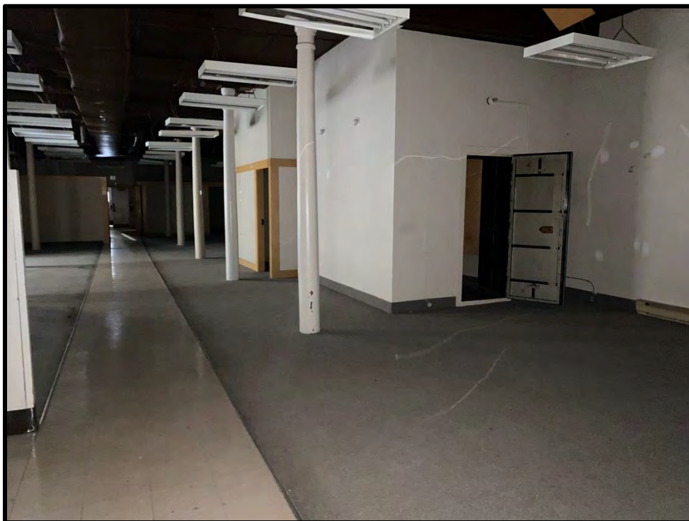
Image 80: First Floor North Addition – Interior (Photo taken on December 8, 2021; Facing West)
