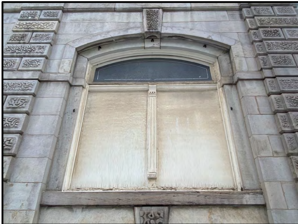
Image 26: East Elevation Window Opening - Detail (Photo taken on December 8, 2021; Facing West)
