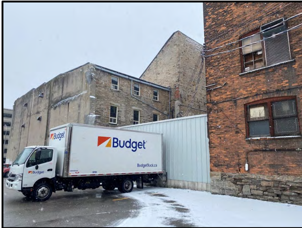
Image 17: West Elevation (Photo taken on December 8, 2021; Facing Southeast)
