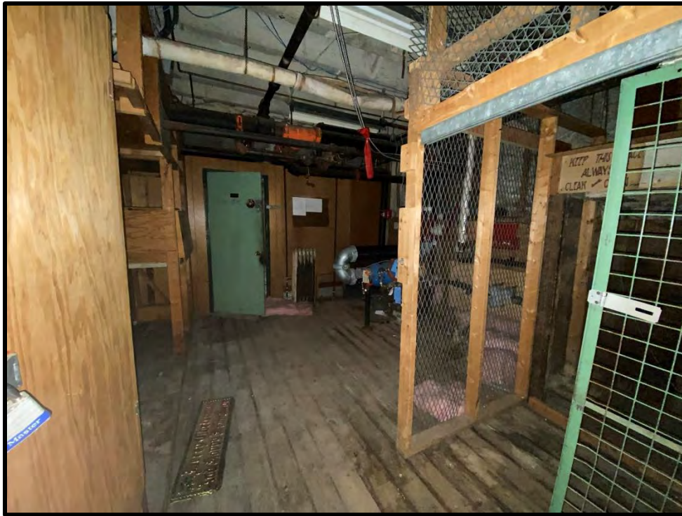
Image 187: Basement Brick Building – Interior (Photo taken on December 8, 2021)
