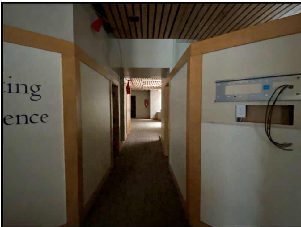
Image 66: First Floor – Interior (Photo taken on December 8, 2021; Facing North)
