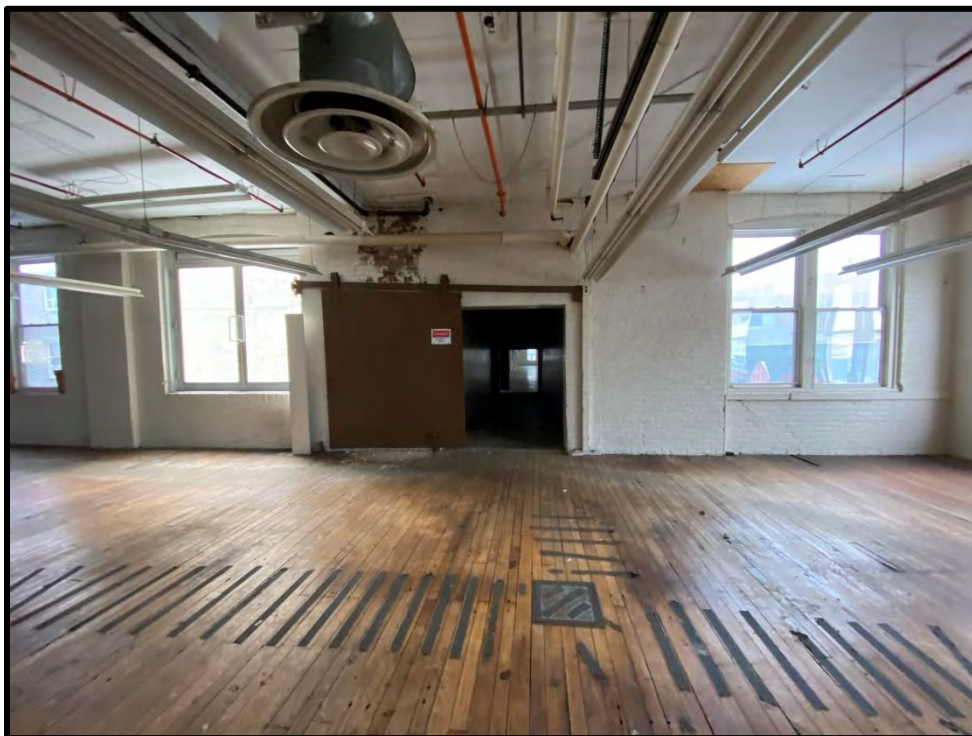
Image 170: Second Floor Brick Building – Opening to Stone Building (Photo taken on December 8, 2021; Facing East)
