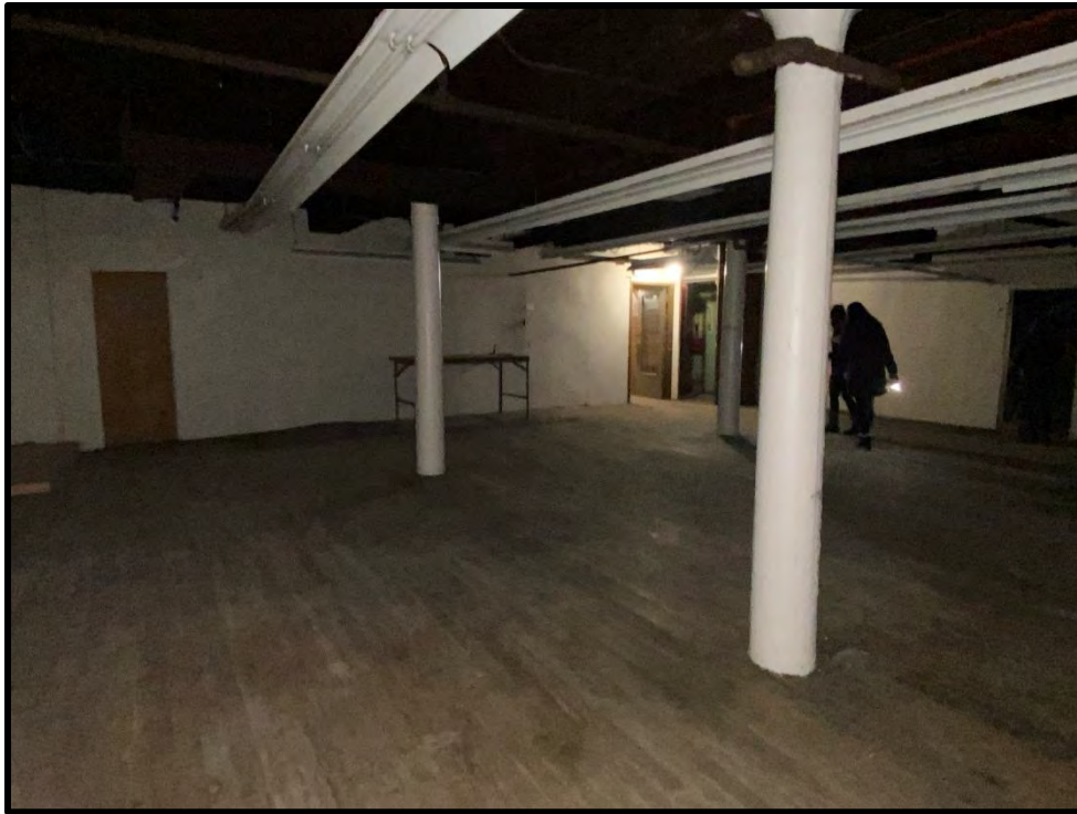
Image 145: Basement Stone Building – Interior (Photo taken on December 8, 2021)
