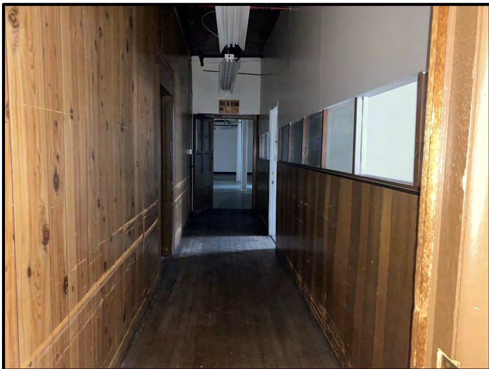
Image 118: Second Floor North Addition – Interior (Photo taken on December 8, 2021; Facing South)
