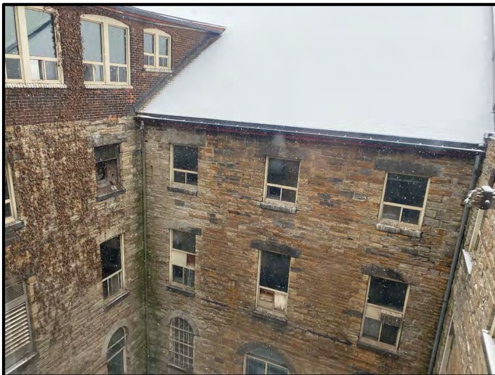
Image 32: Courtyard (Photo taken on December 8, 2021; Facing Southwest)
