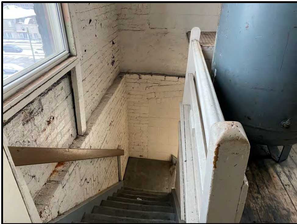
Image 174: Third Floor Brick Building – Stairwell (Photo taken on December 8, 2021; Facing Northeast)
