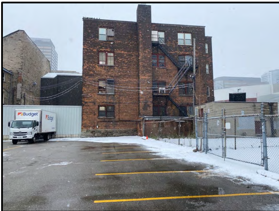
Image 50: North Elevation (Photo taken on December 8, 2021; Facing South)
