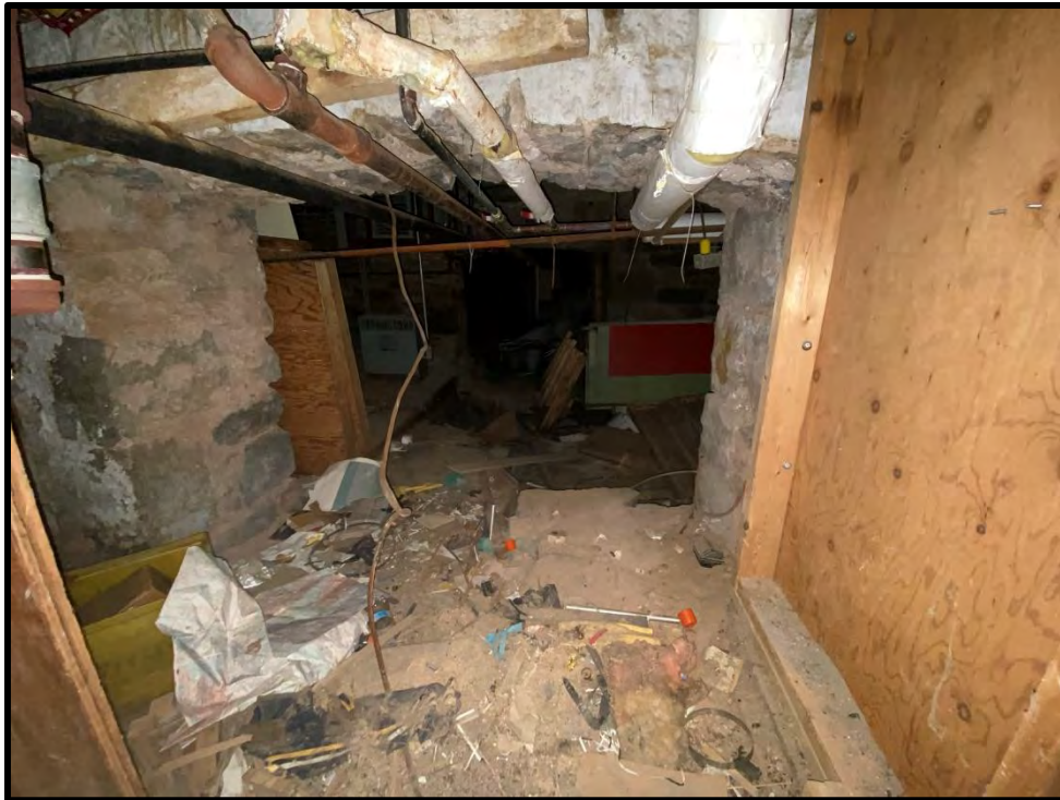
Image 147: Basement Stone Building – Interior (Photo taken on December 8, 2021)
