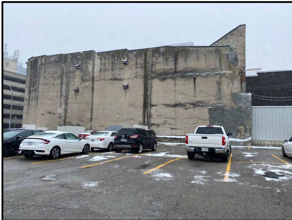
Image 18: North Elevation (Photo taken on December 8, 2021; Facing South)
