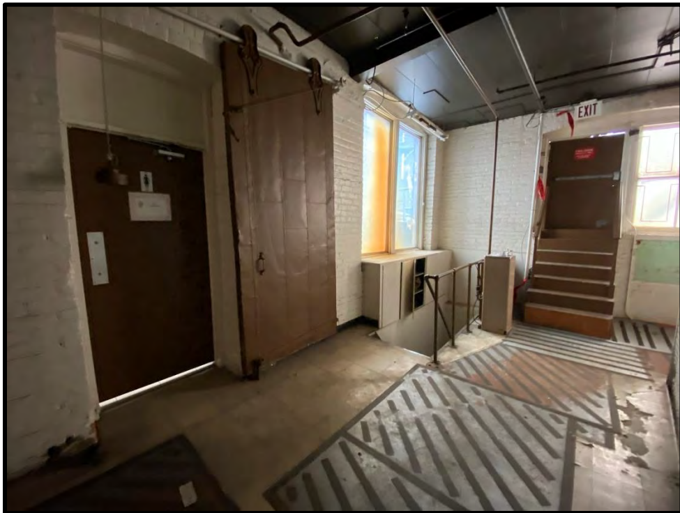
Image 166: First Floor Brick Building – Interior (Photo taken on December 8, 2021; Facing Northeast)
