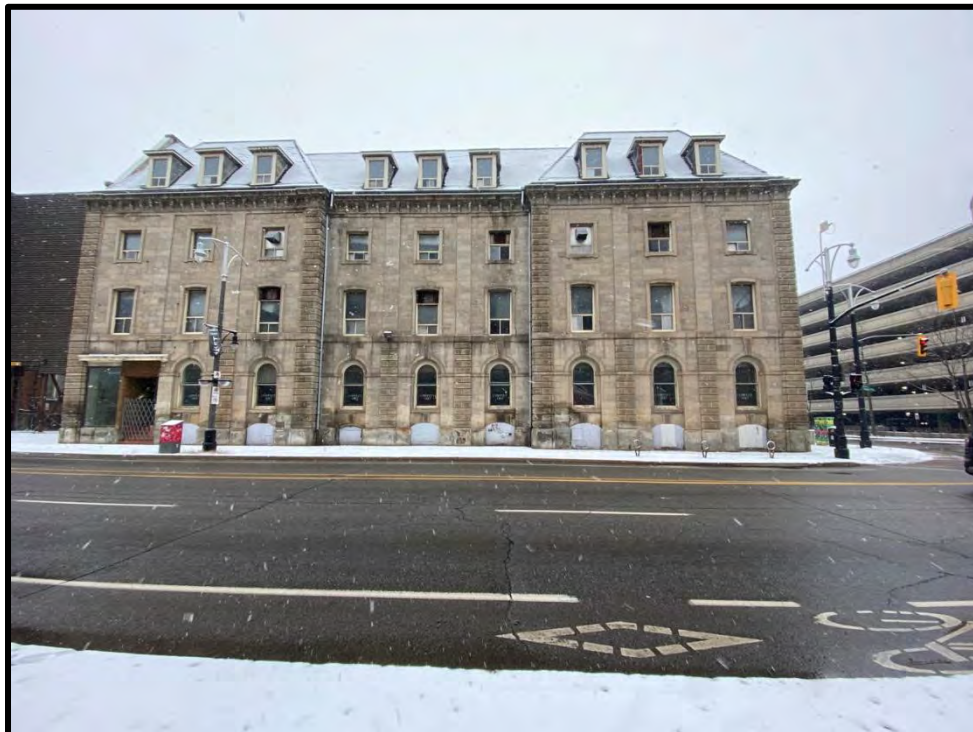
Image 4: York Street Front Façade (South Elevation) (Photo taken on December 8, 2021; Facing North)
